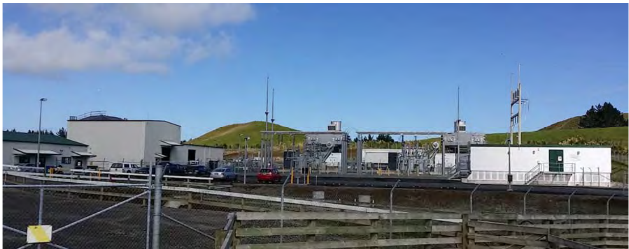
Photo 1 Nova McKee Power Plant
