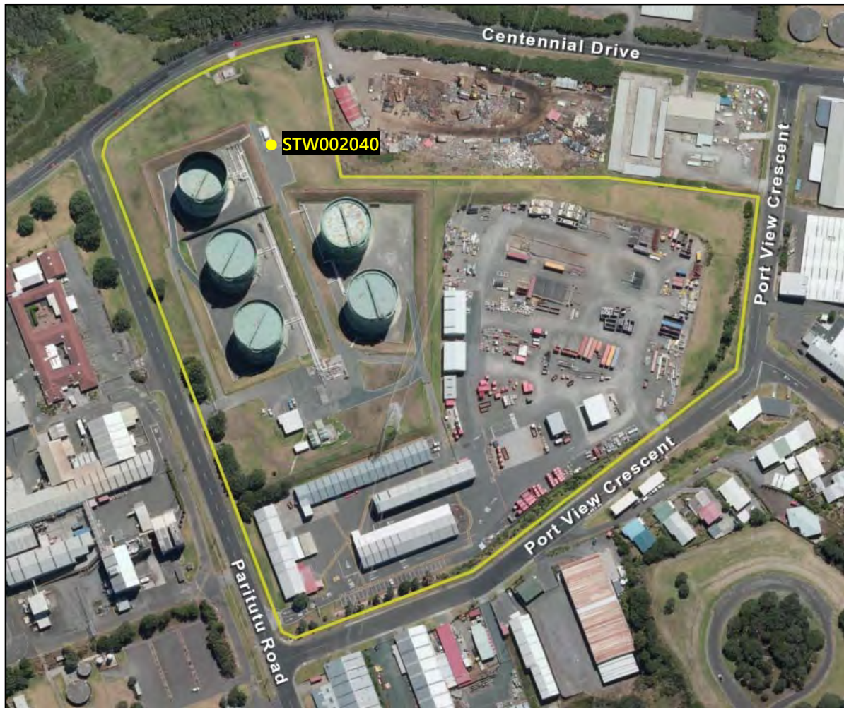
Figure 6 Aerial photograph of the STOS Paritutu Tank Farm
