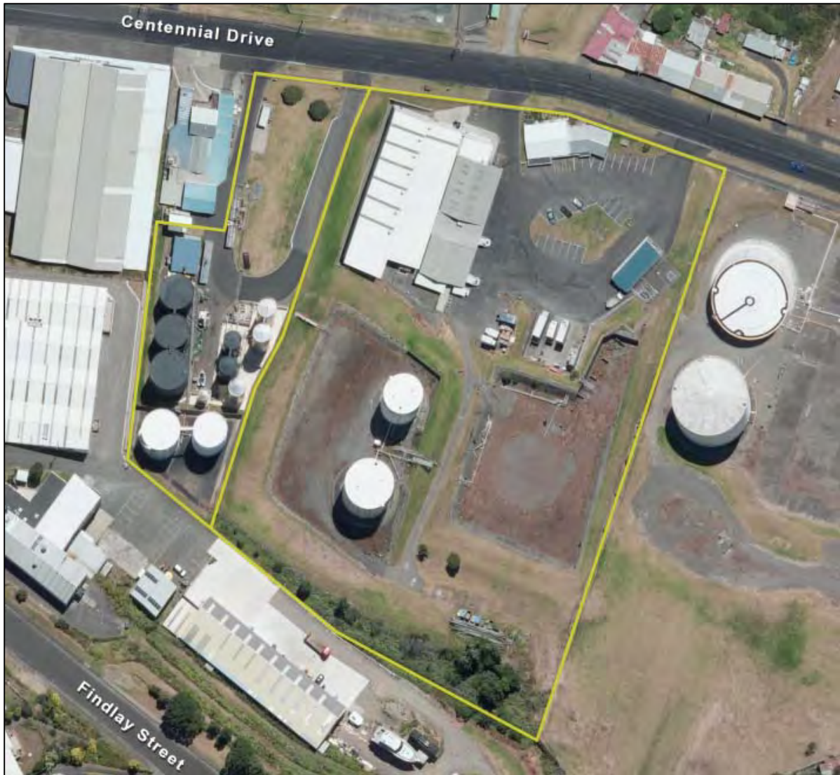
Figure 2 Aerial photograph of the Bulk Storage Terminals Ltd site
