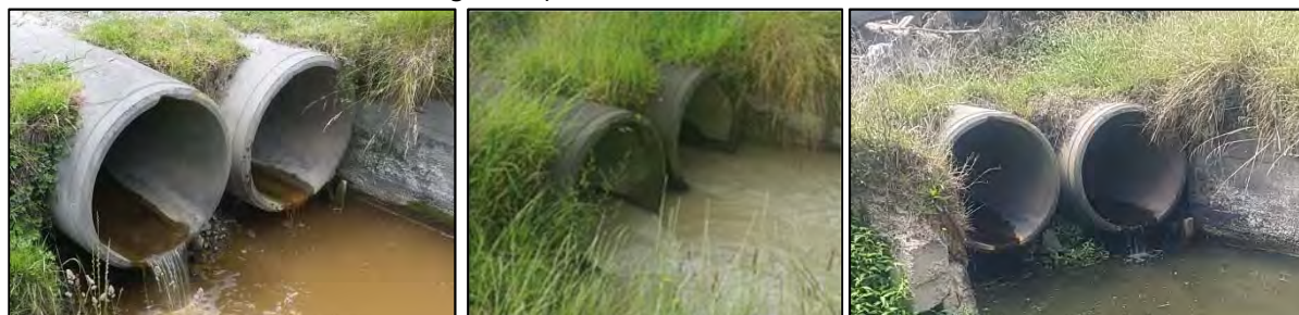
Photo 2 The access culvert immediately upstream of site 2, December 2015 (left), December 2016 (middle) and January 2018 (right).
