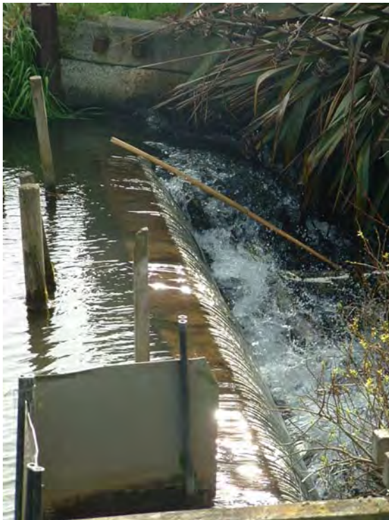
Photo 1 The weir and fish pass on the Tawhiti Stream (fish pass visible on far side)
