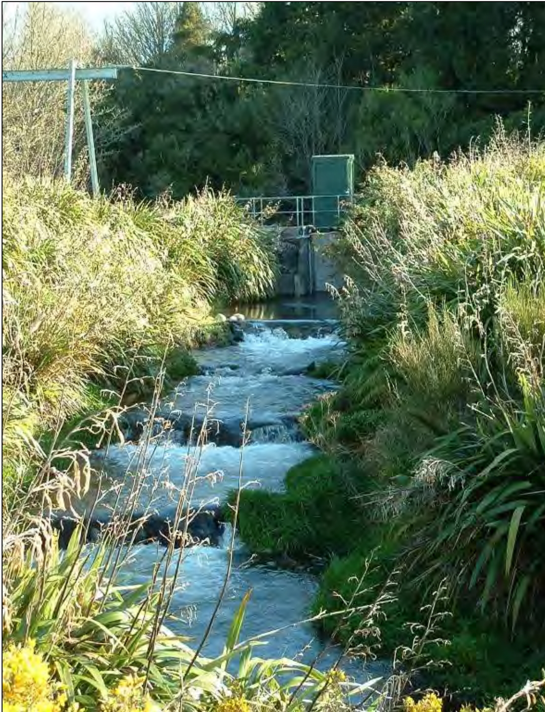
Photo 1 The new fish pass, 8 September 2010
