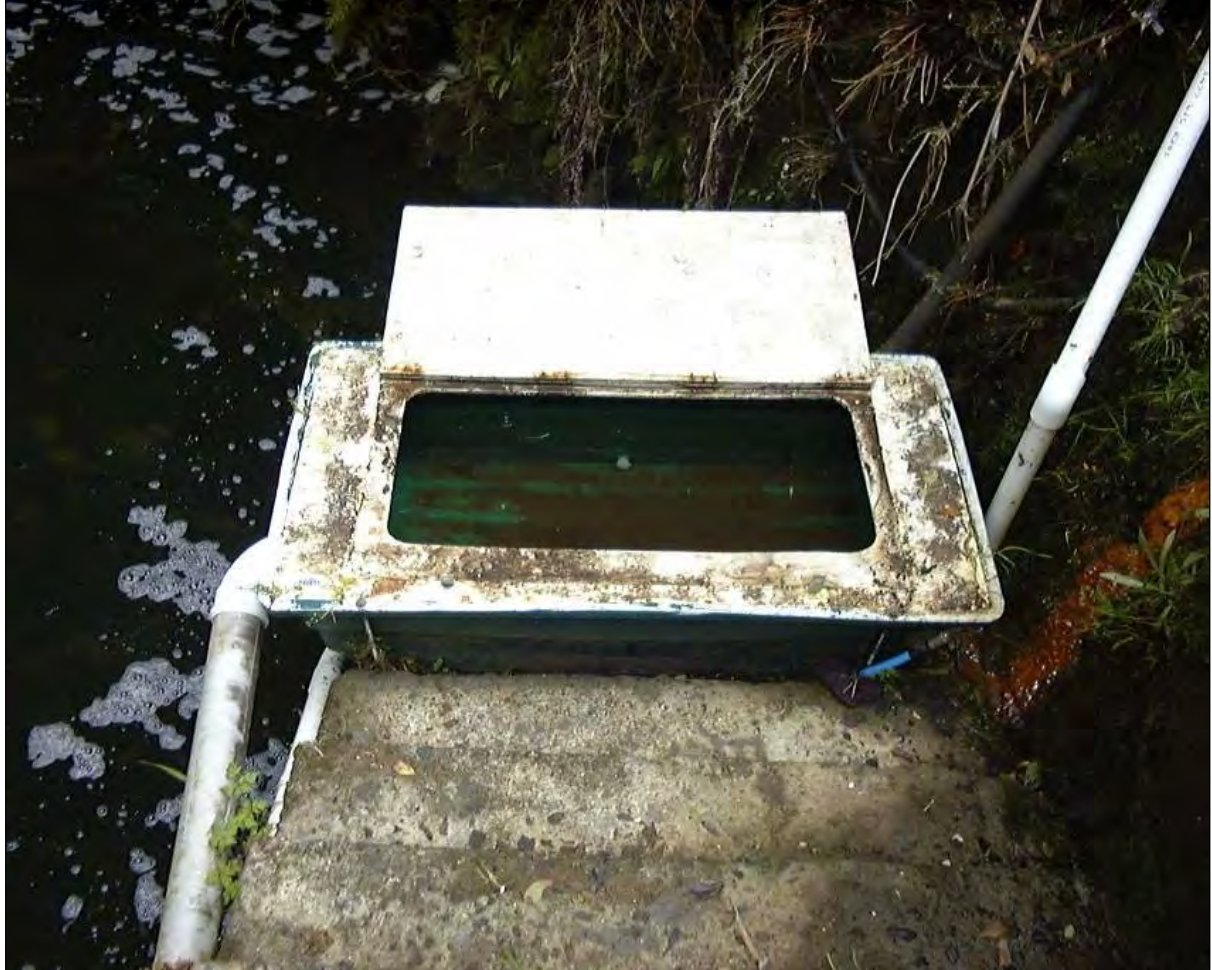
Photo 7 Elver trap at the base of the tail race at the power station, prior to upgrade
