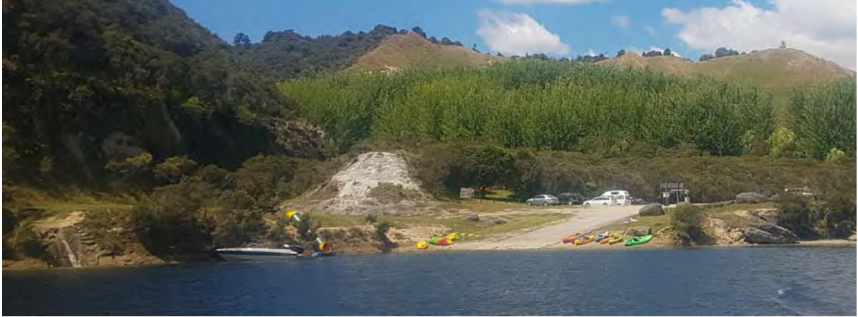
Photo 2 Patea Dam boat ramp, 15 February 2018
