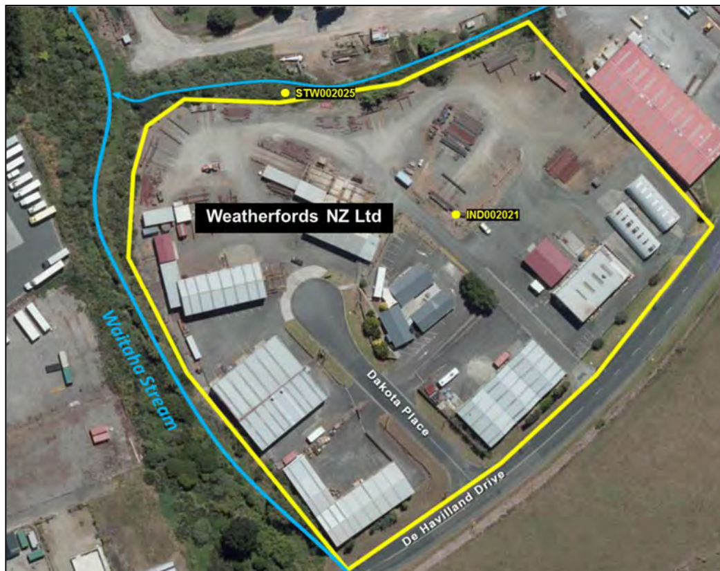
Figure 16 Aerial view of Weatherford's site
