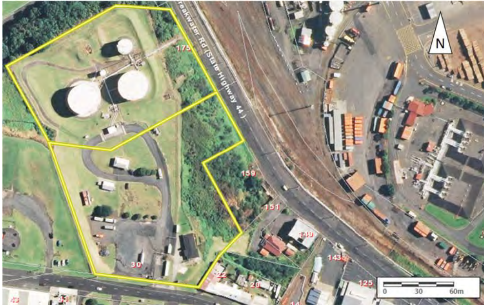
Figure 3 Aerial photograph of the New Zealand Oil Services Ltd Centennial Drive site
