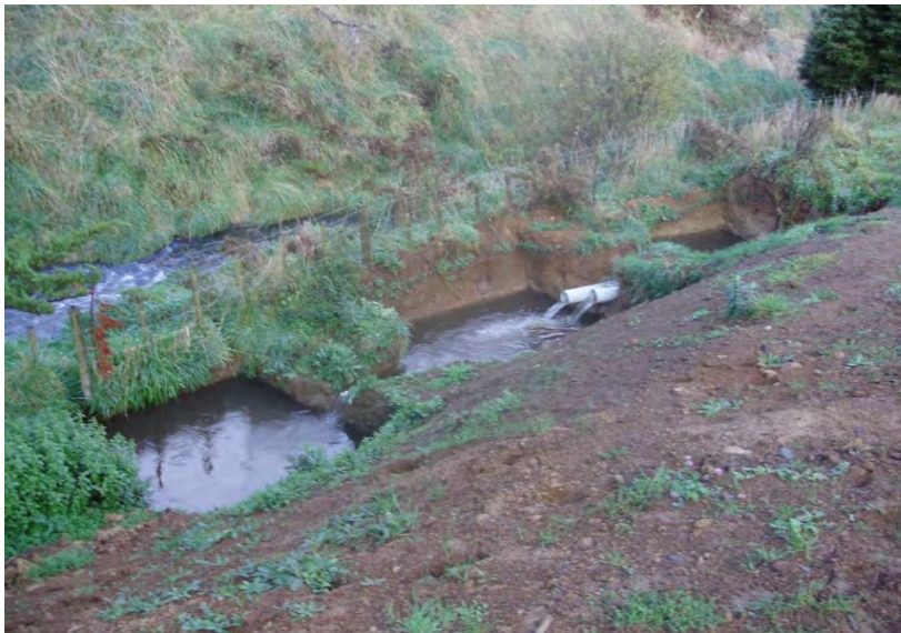
Photo 2 The settling system at Taranaki Fish and Game trout hatchery
