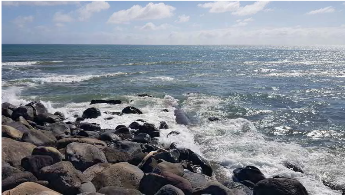
Photo 1 Outfall pipe during the 2017-2018 backwash inspection (4 April 2018)
