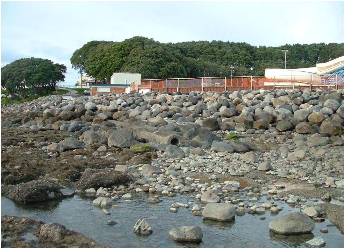
Photo 1 Aquatic Centre ocean outfall
