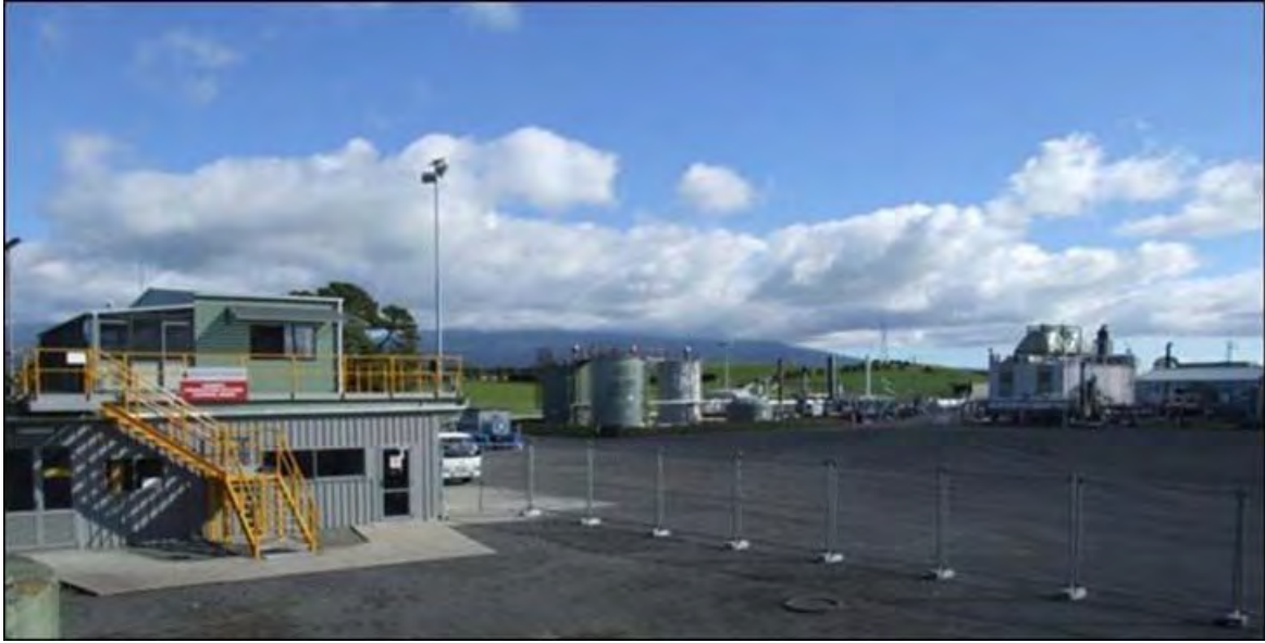
Photo 1 Kaimiro Production Station
