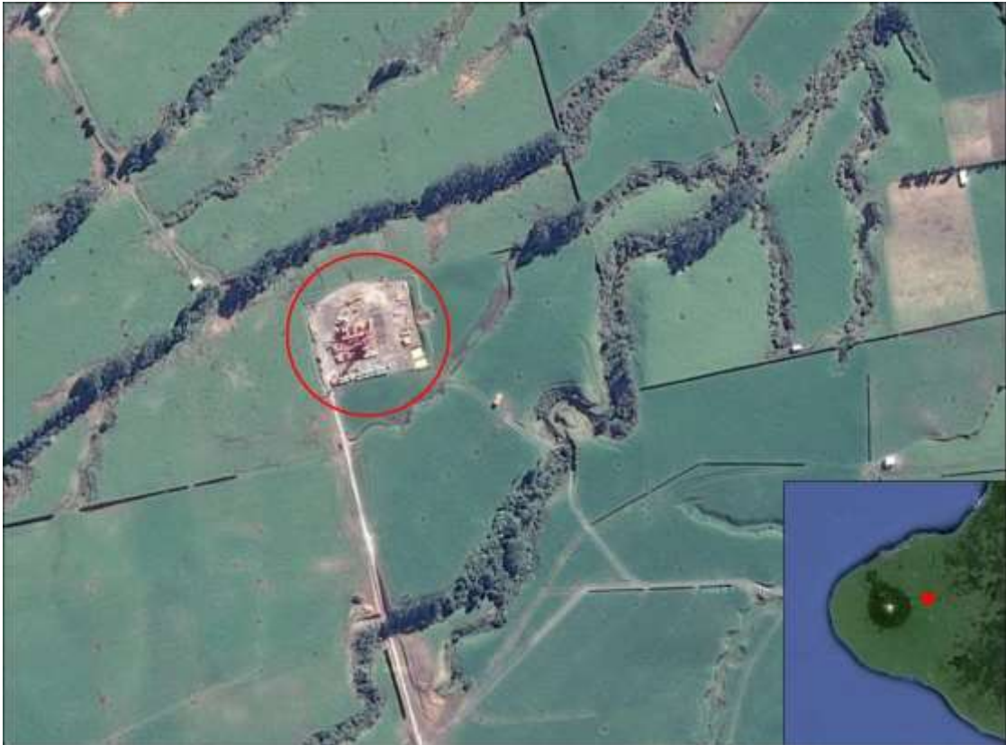
Figure 1 Aerial view depicting the locality of the York-A wellsite, with approximate regional location (inset)
