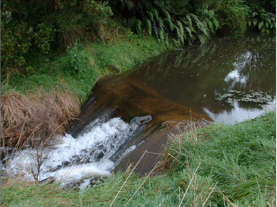
Photo 2 McKee Production Station water supply weir in the Mangaheua Stream
