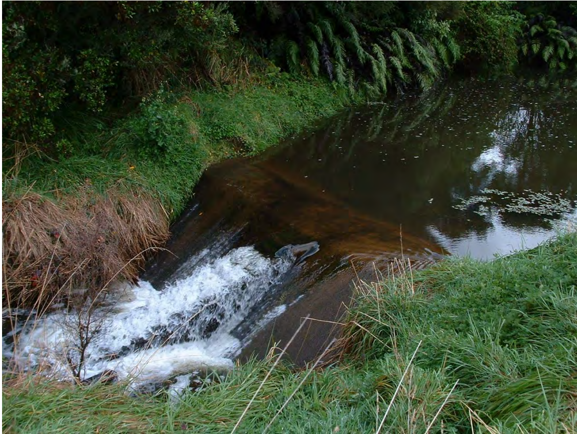
Photo 1 McKee Production Station water supply weir in Mangahewa Stream, with the fish pass in the centre of the weir.
