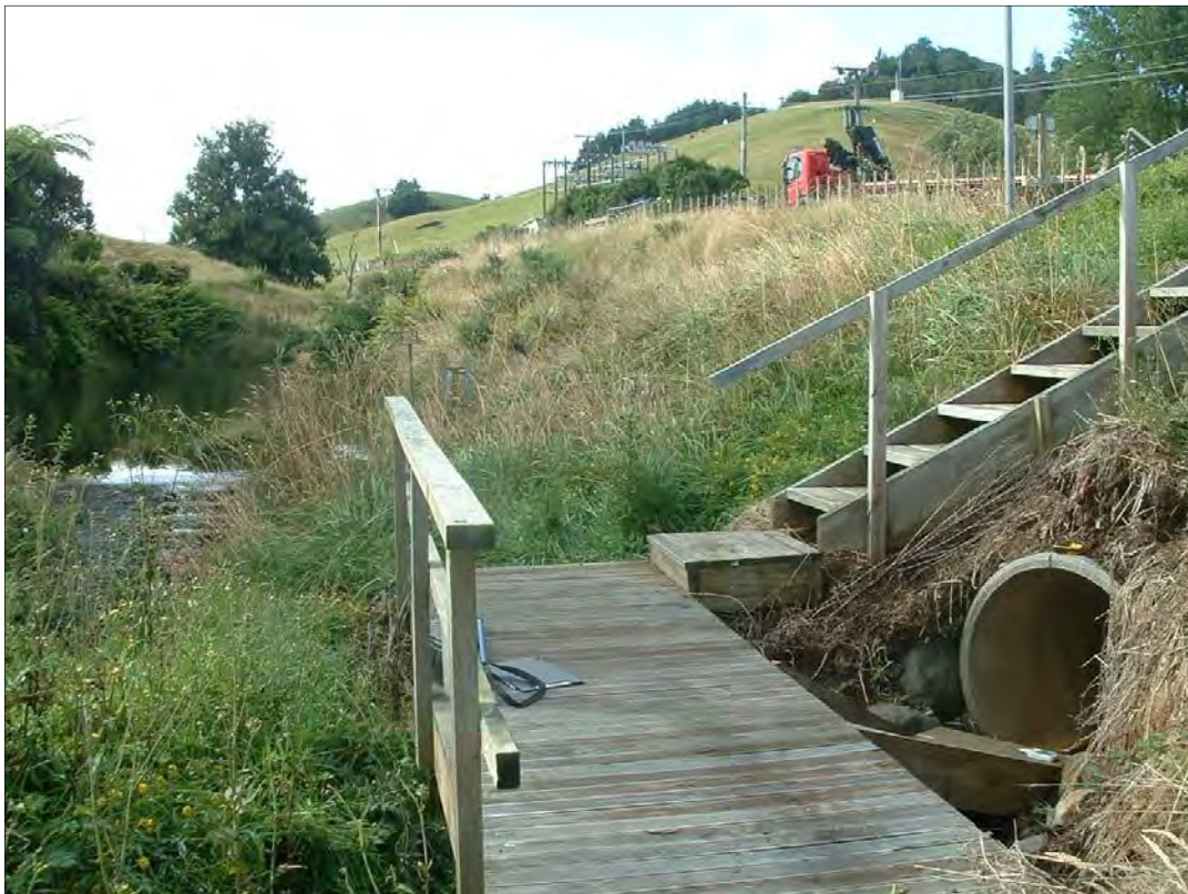
Photo 3 McKee Production Station stormwater discharge to the Mangahewa Stream
