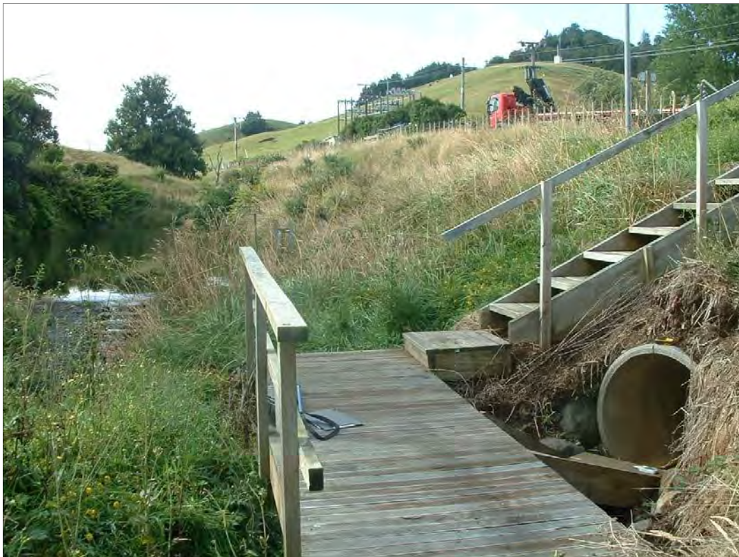
Photo 2 McKee Production Station stormwater discharge to the Mangahewa Stream
