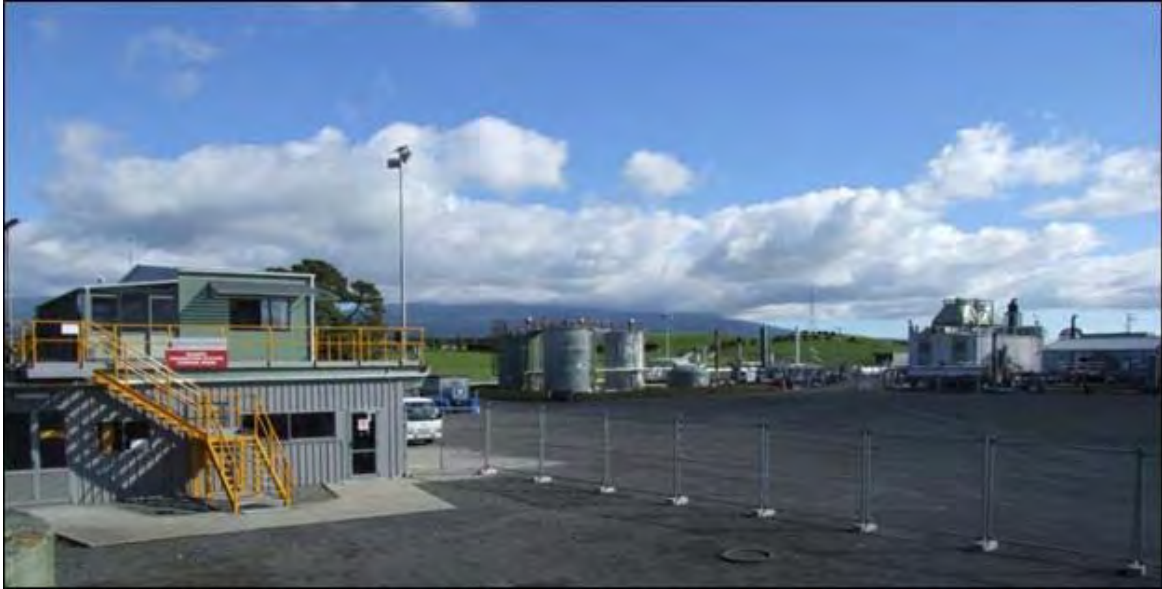
Photo 1 Kaimiro Production Station
