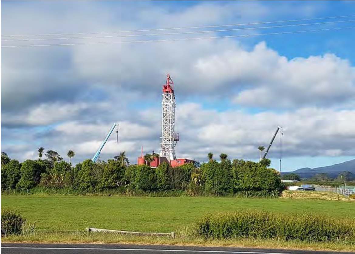
Photo 2 Radnor Production Station
