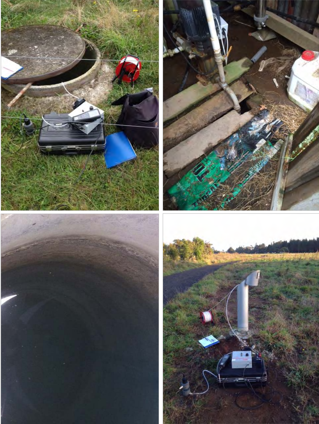
Photo 1 Various examples of well construction types in Taranaki. Top left: Dug and lined well GND1098, Top right: Dug - unlined well GND1082, Bottom left: Example of internal well lining in dug well GND1095, Bottom right: drilled and screened well GND2484 (being sampled with a peristaltic pump).
