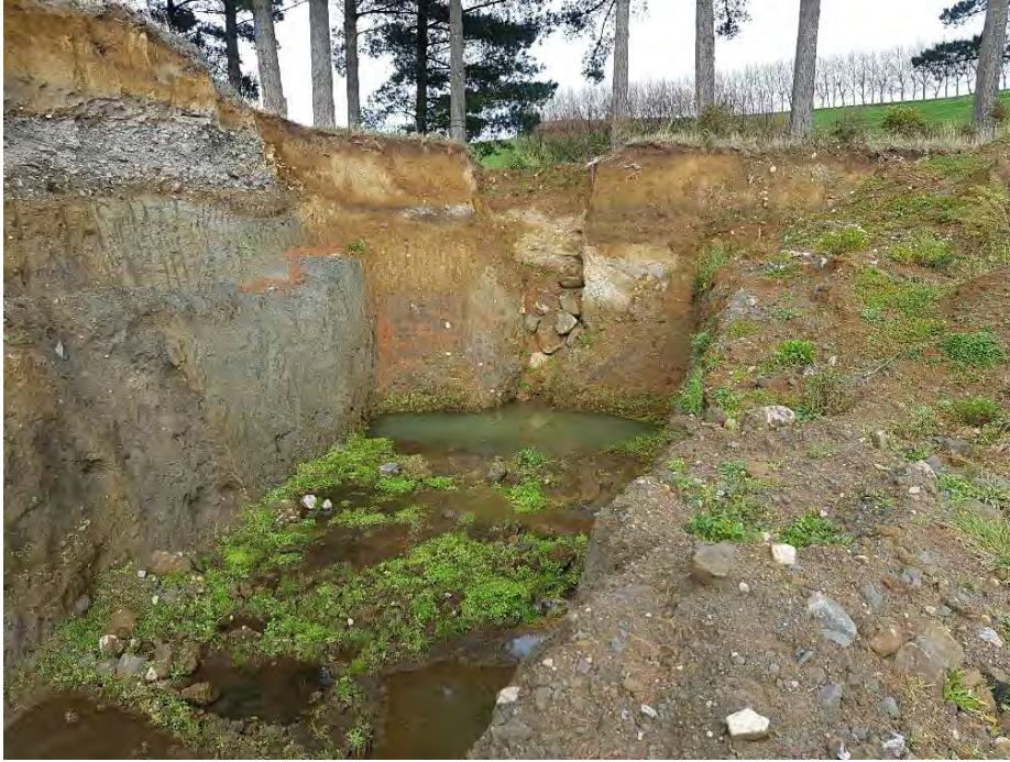
Photo 9 Discharge point from excavation pit
