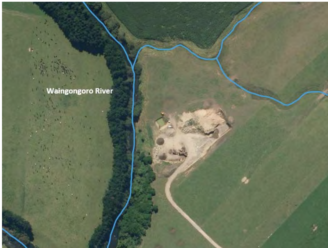
Figure 13 Horizon Trust Management Limited Whenuku Road quarry
