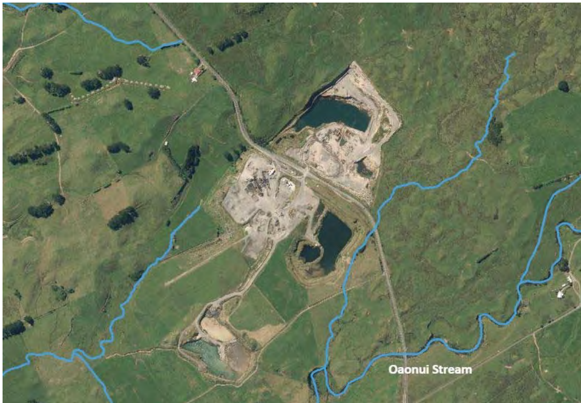
Figure 10 Wiremu Road Quarry Limited quarry site
