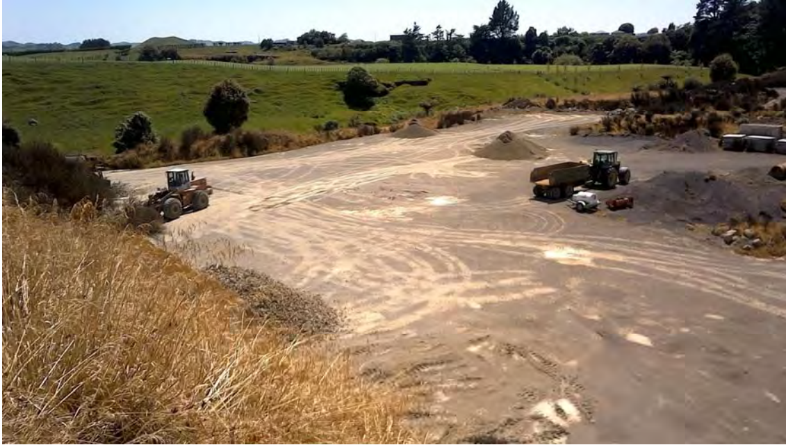
Photo 12 Taunt Contracting Limited Quarry site
