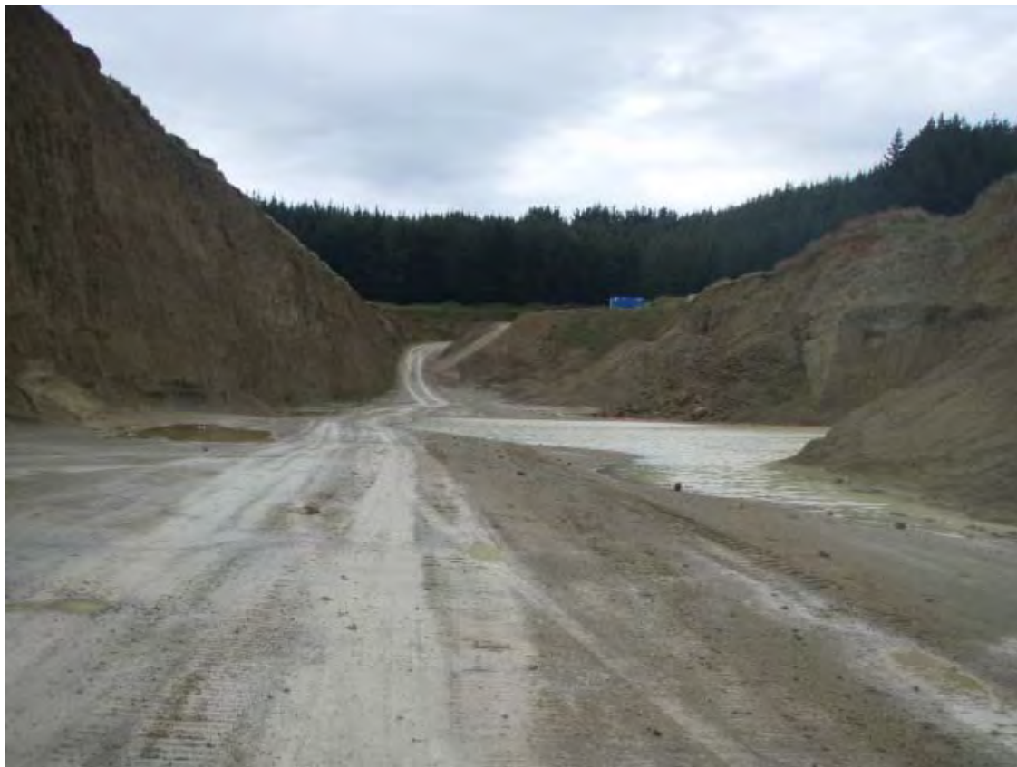
Photo 13 Stormwater collection area at base of quarry pit from which stormwater drains via seepage to ground
