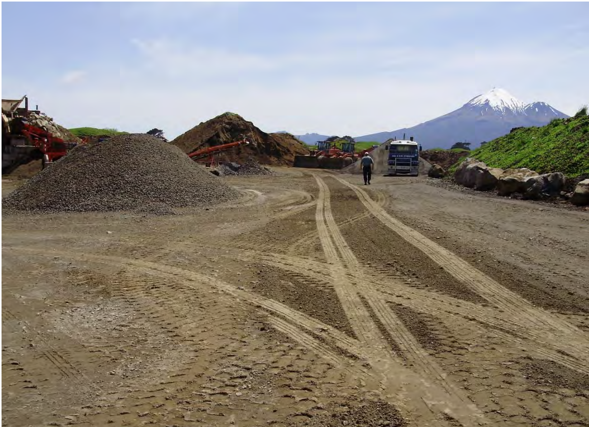
Photo 8 Waiteika Road quarry site 2009
