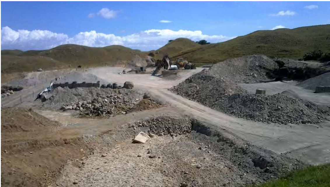
Photo 3 Goodin AG Limited quarry site
