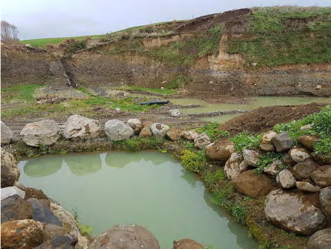
Photo 7 Bunded pooled section of the tributary
