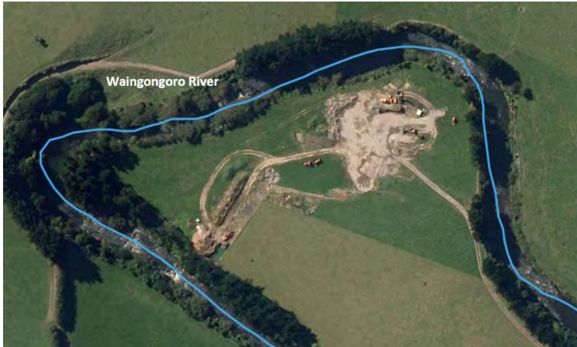
Figure 15 Bourke Quarry site
