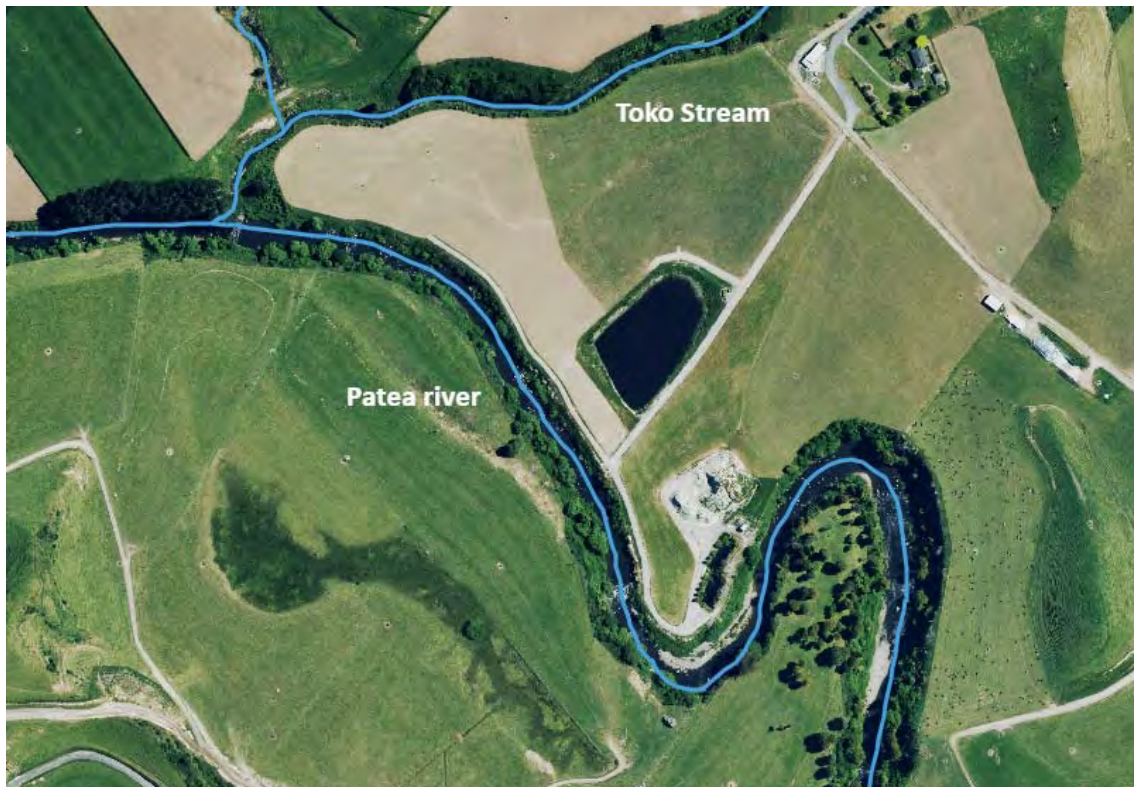
Figure 16 Vickers Quarries Limited Toko Road quarry site
