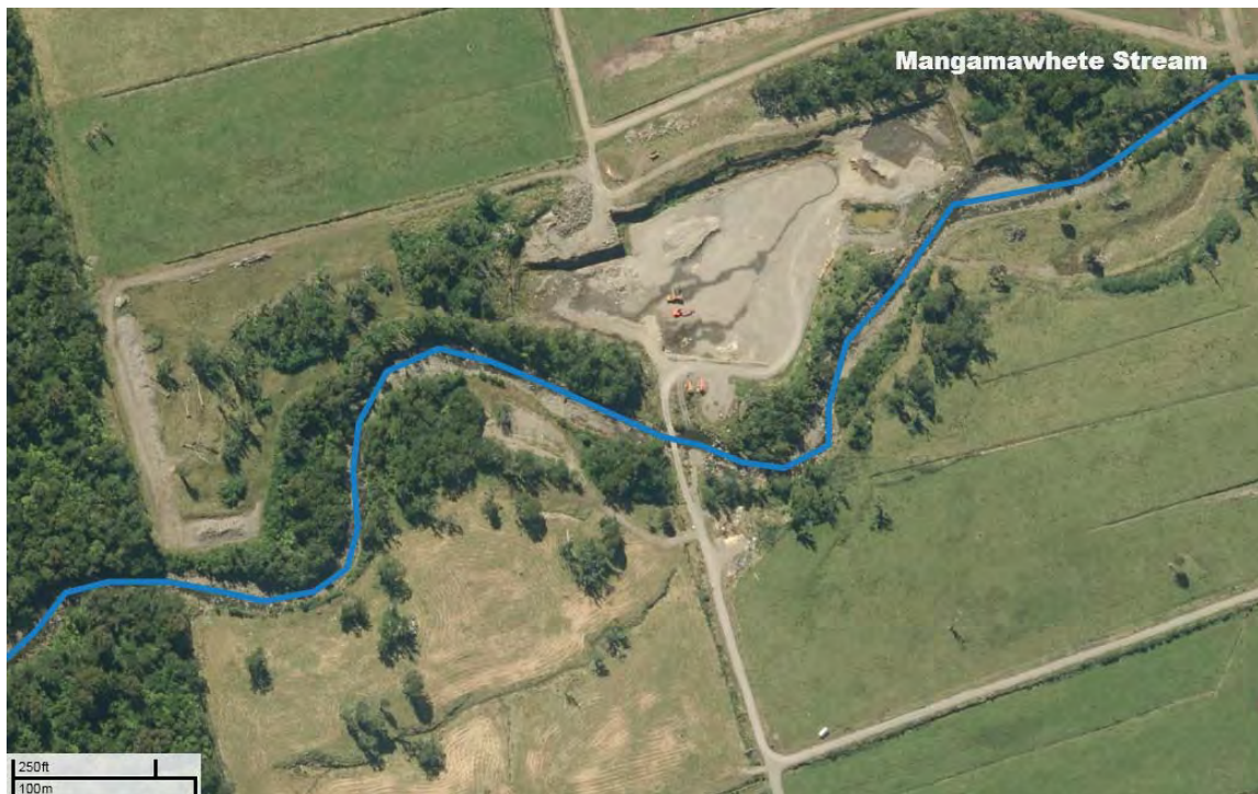
Figure 5 C D Boyd Surrey Road quarry site
