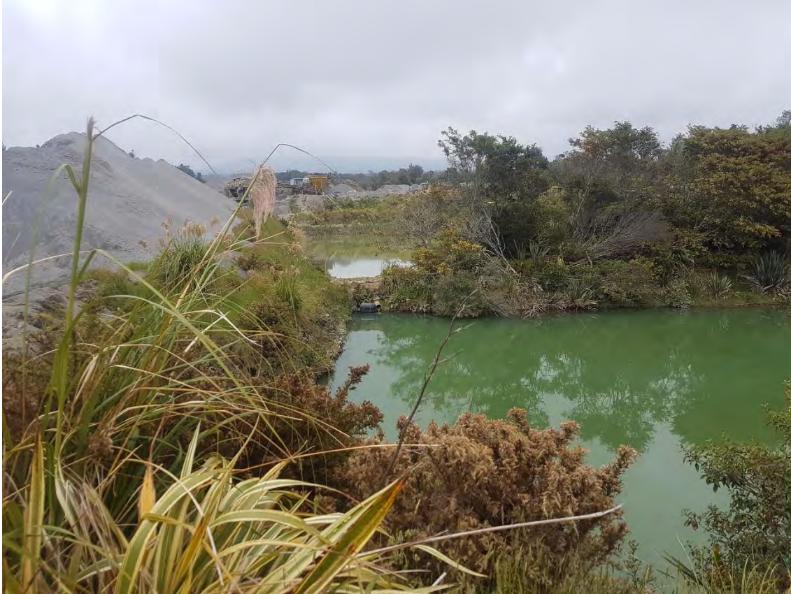
Photo 14 Vickers Quarries Limited York Road settlement ponds 27 November 2017
