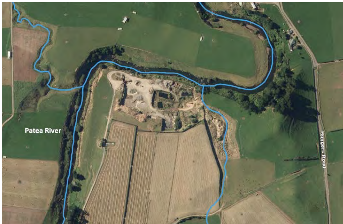
Figure 14 Taunt Contracting Limited Bird Road quarry site
