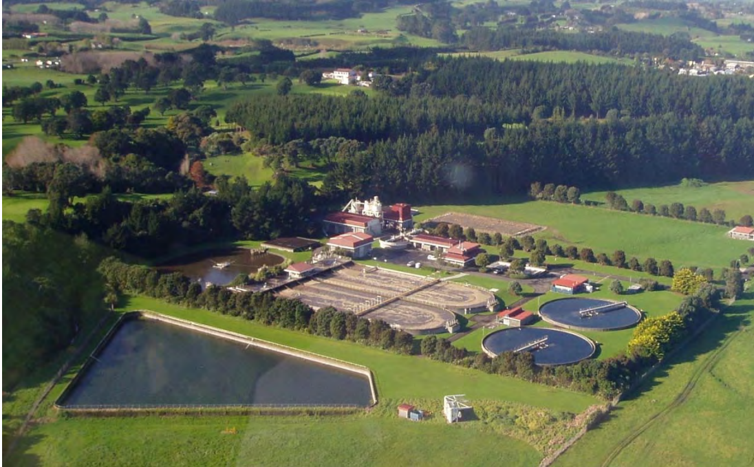
Photo 1 The New Plymouth Wastewater Treatment Plant
