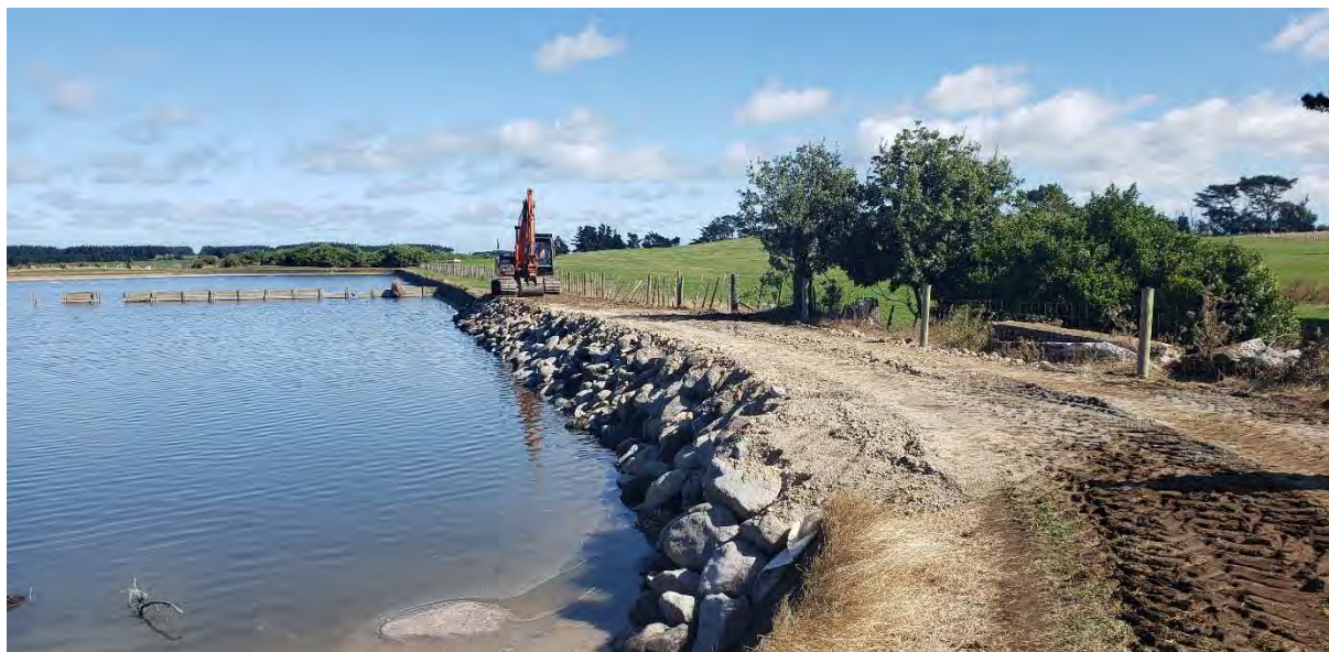
Photo 10 Repairs to Waverley WWTP wave band, April 2019
