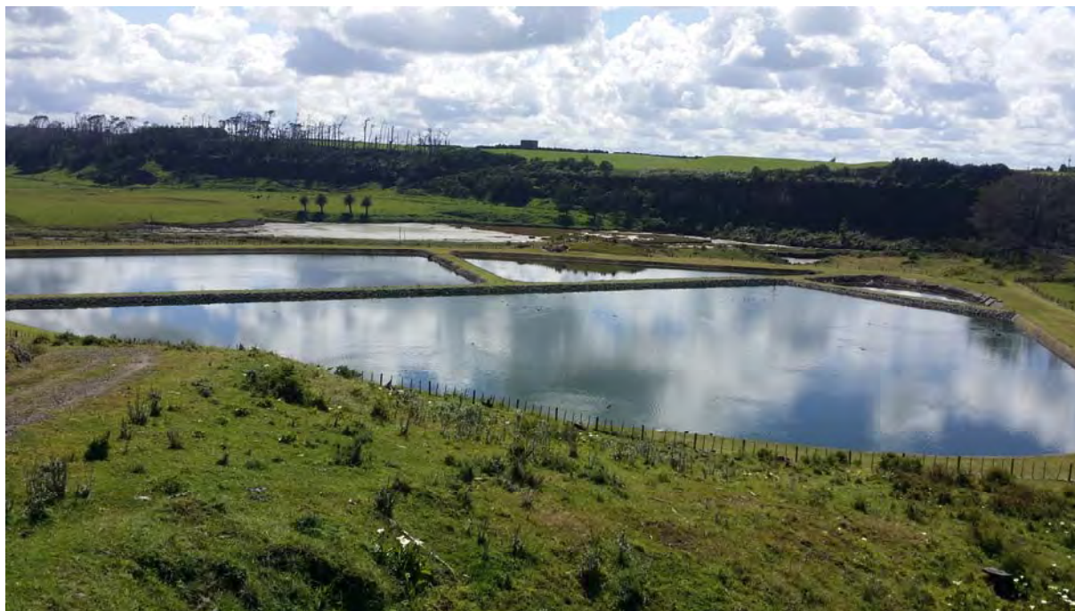
Photo 7 View of Patea WWTP
