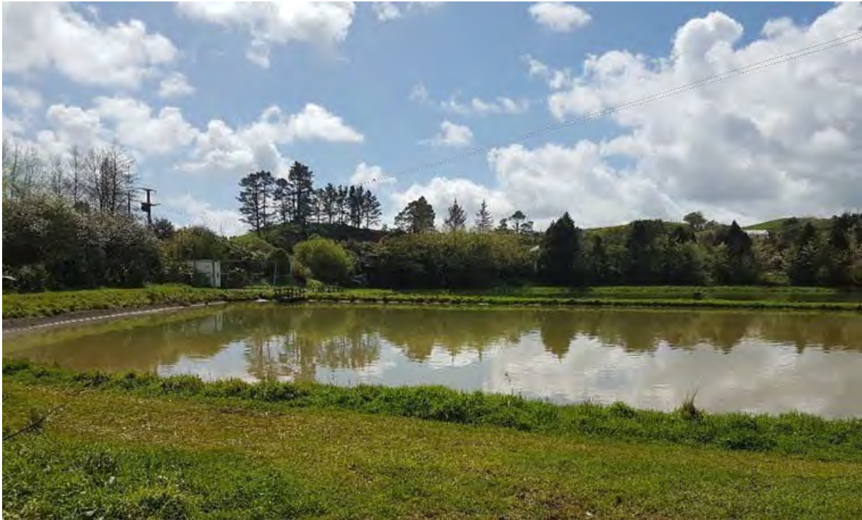
Photo 2 The Inglewood WWT main pond
