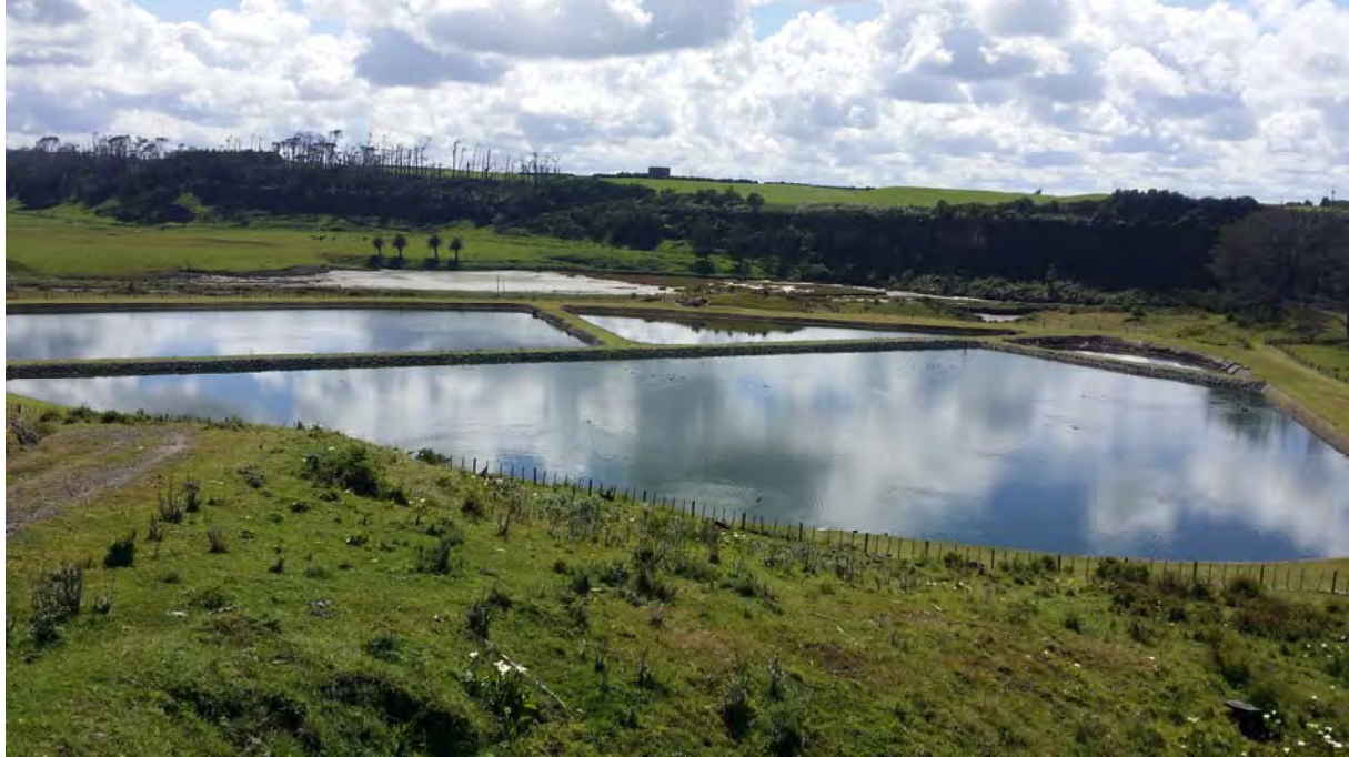
Photo 7 View of Patea WWTP
