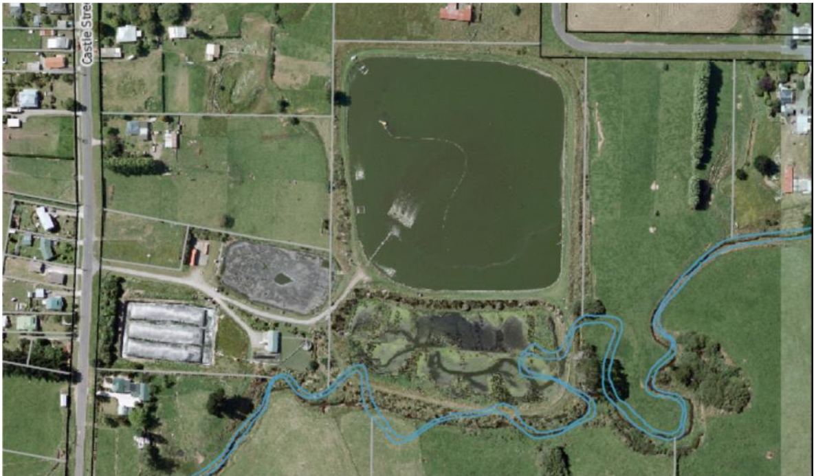
Figure 2 Aerial view of the Eltham WWTP showing the sludge geo-textile bags disposal area (lower LH corner) near the plant entrance [Note: the wetland (lower, centre) was converted to a holding pond in early 2011]
