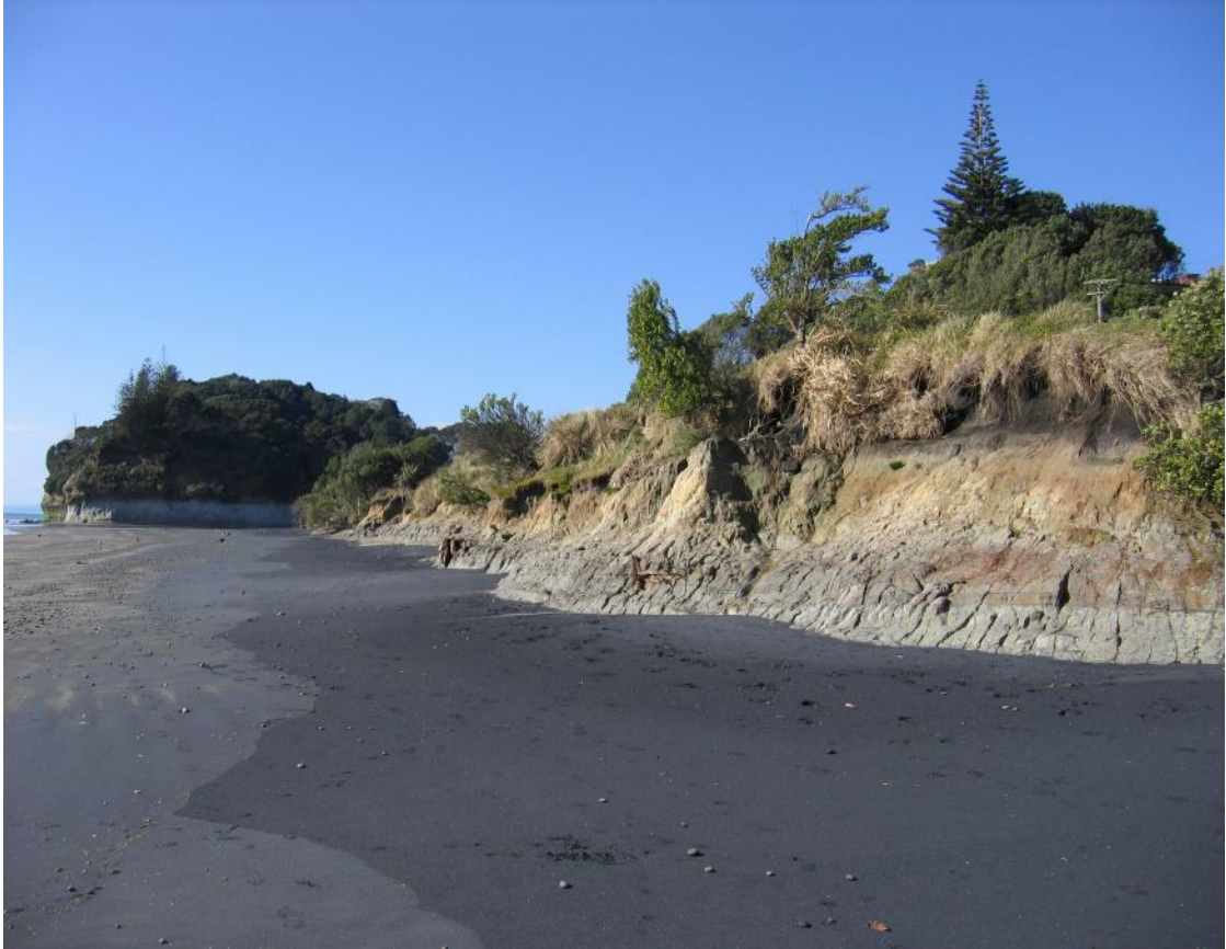
Photograph 3 Erosion on Wai-iti foreshore prior to construction of the rock rip rap seawall
