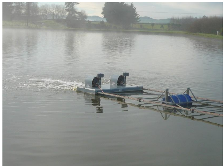
Photo 2 Replacement aerator, June 2013
