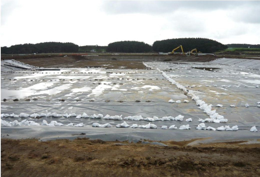
Photo 1 Construction of maturation ponds, July 2009
