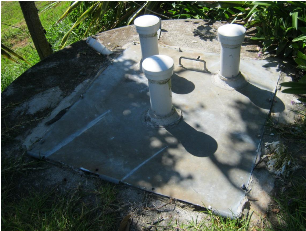
Photo 3 Pump station lid (29 January 2013)
