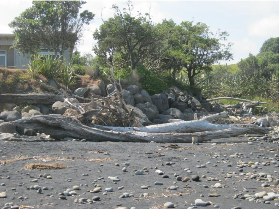
Photograph 7 Tree trunks placed at the stream mouth to reduce erosion
