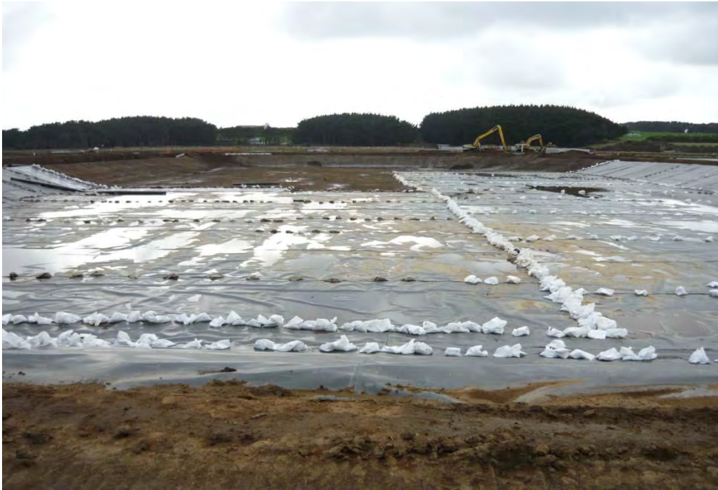
Photo 1 Construction of maturation ponds, July 2009
