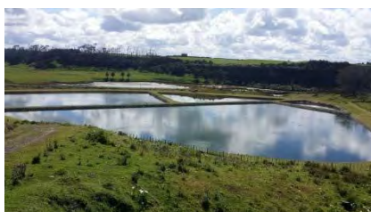
Photo 144 General view of three cell system November 2014
