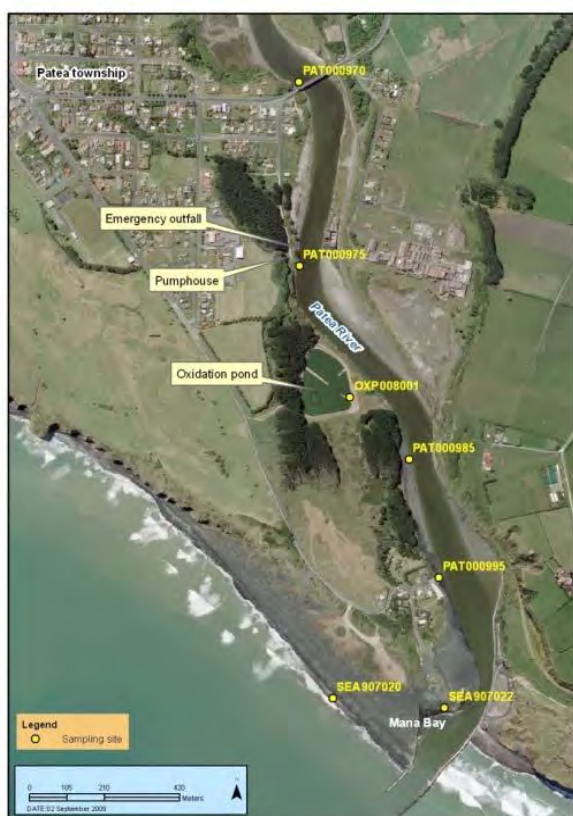
Figure 7 Aerial location map of sampling sites in relation to the Patea upgraded three cell oxidation pond system
