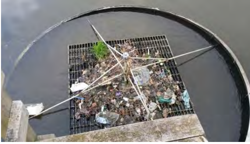
Photo 1 & 2 Primary pond outlet, December 2014 and June 2015
