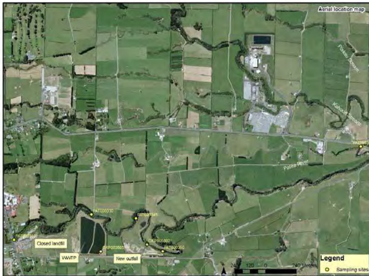
Figure 1 Aerial photo of site and location of sampling sites since the upgrade of the WWTP
