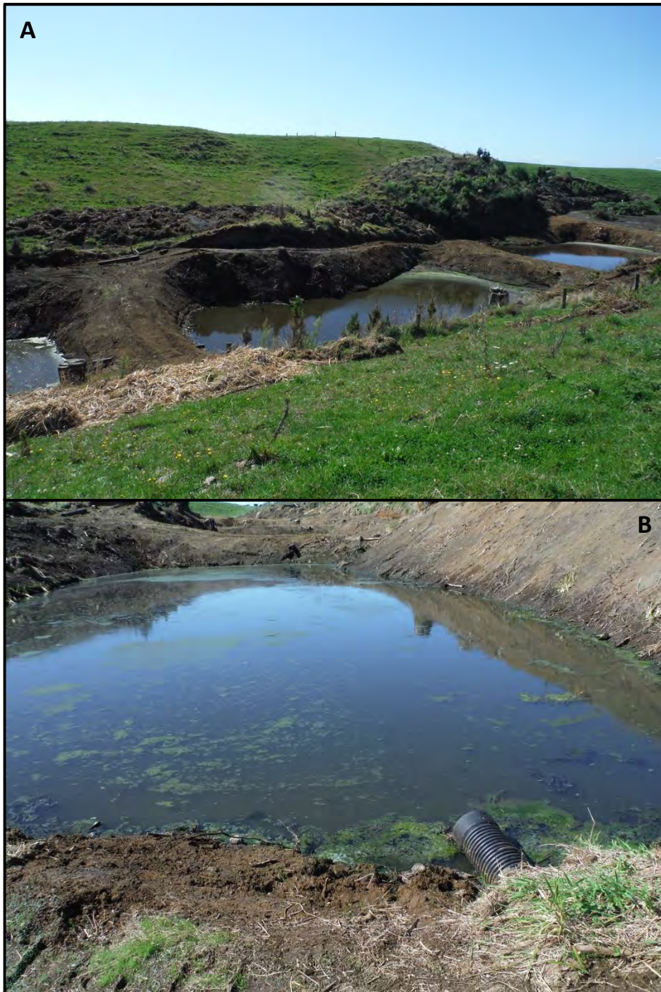
Photo 3 A) Three pond dairy effluent system B) Final pond with discharge pipe
