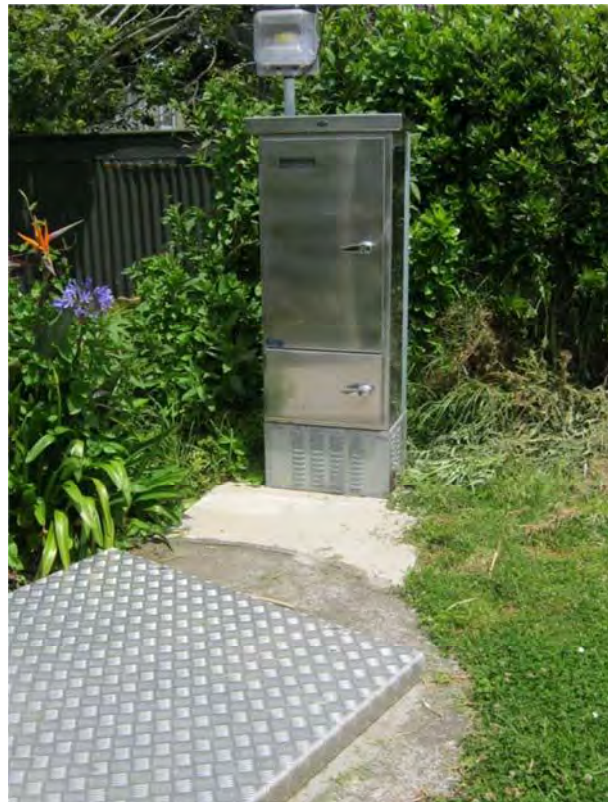
Photo 4 Onaero pump station (16 December 2014)
