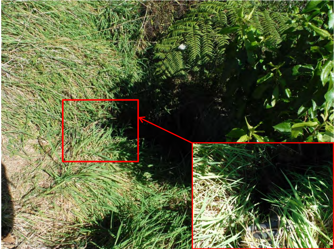
Photo 4 Discharge pipe (inset) and receiving tributary
