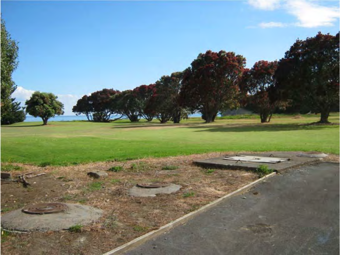
Photo 3 Urenui pump station (8 January 2015)
