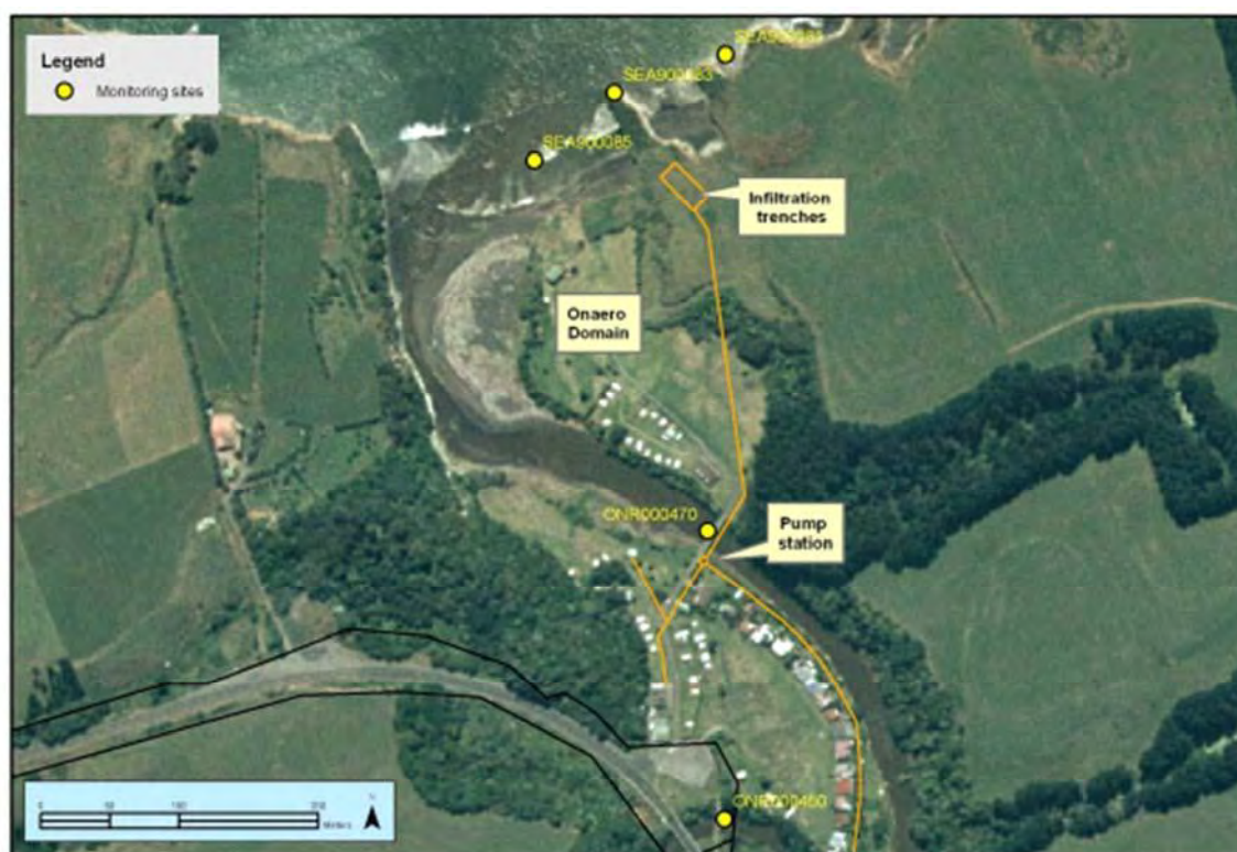
Figure 2 Location of sewage disposal system and sampling sites, Onaero Bay Motor Camp
