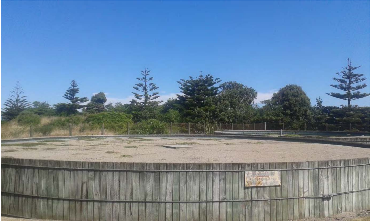
Photo 1 Patchy weed growth on the eastern sand filter (2 March 2015).
