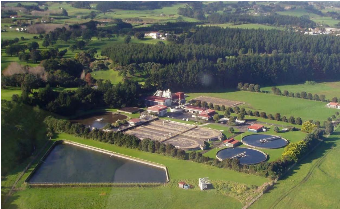
Photo 1 The New Plymouth Wastewater Treatment Plant
