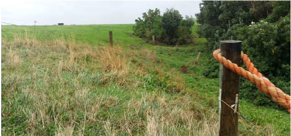
Photograph 2 Fencing around the discharge channel from the oxidation ponds
