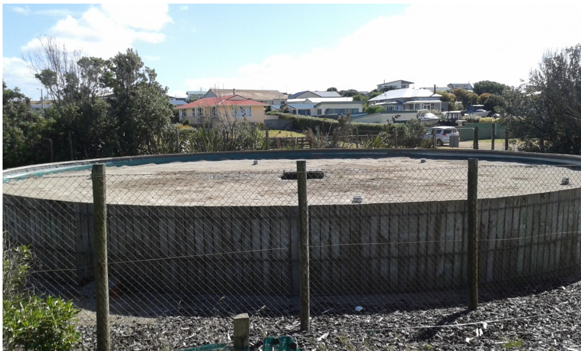
Photo 2 Eastern filter bed with no wastewater ponding or weed growth, 16 February 2016
