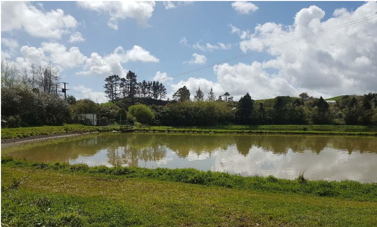
Photo 2 The Inglewood WWTP main pond
