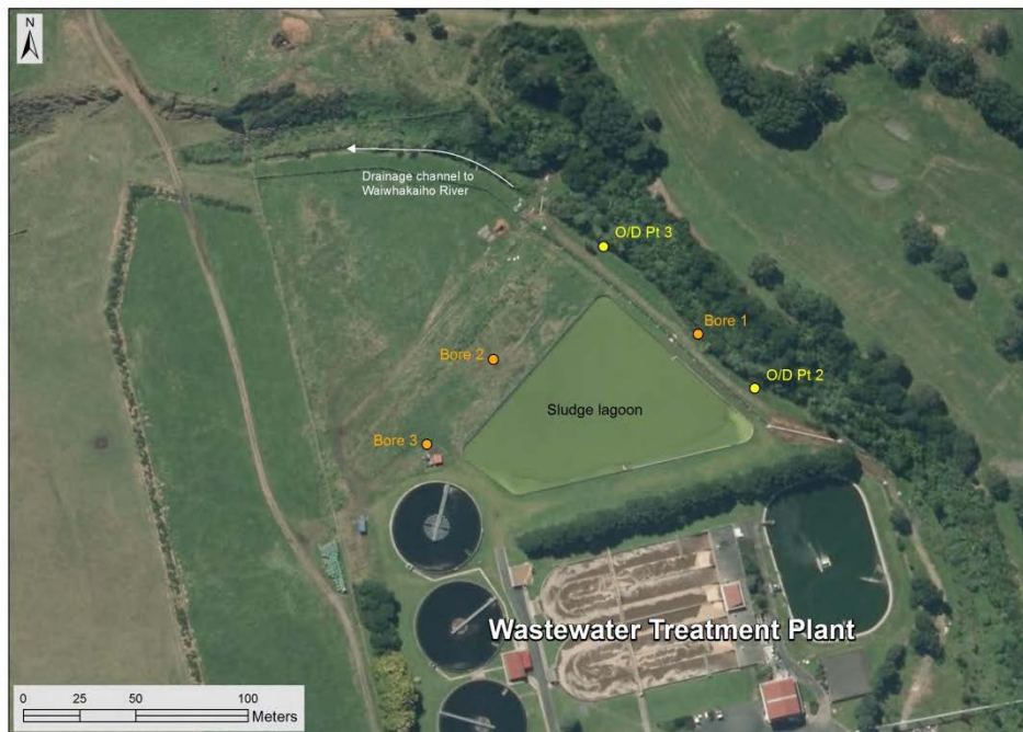
Figure 5 Sludge lagoon showing location of NPDC's groundwater bore and drain sampling sites
