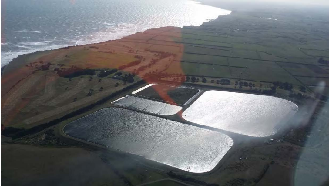
Photo 1 Aerial photograph of the Hawera pond system, 8 March 2016
