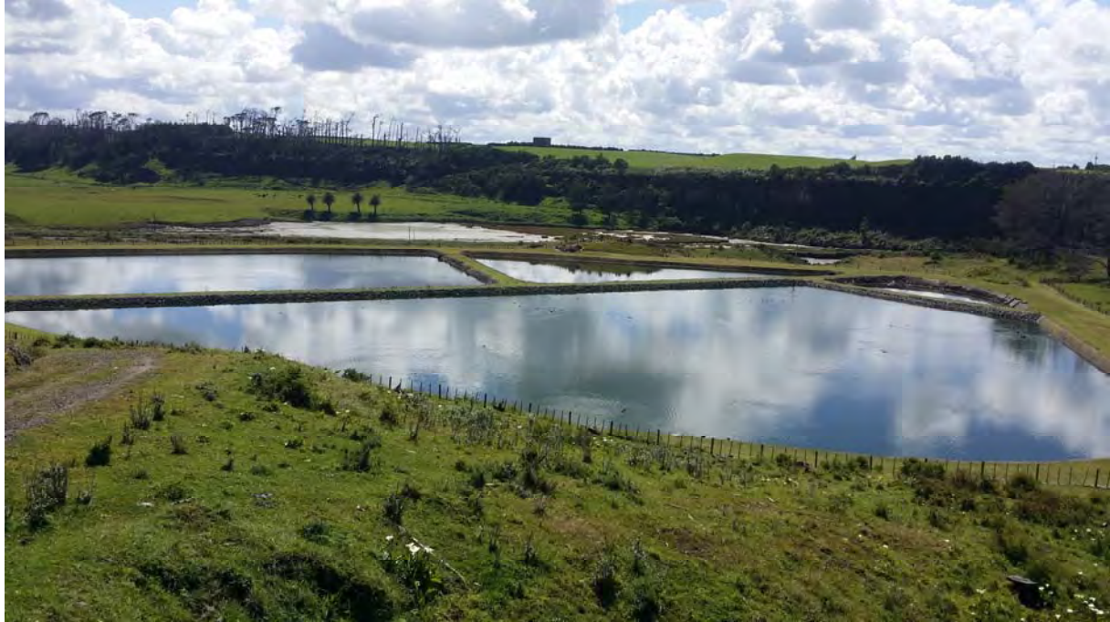
Photo 5 View of Patea WWTP
