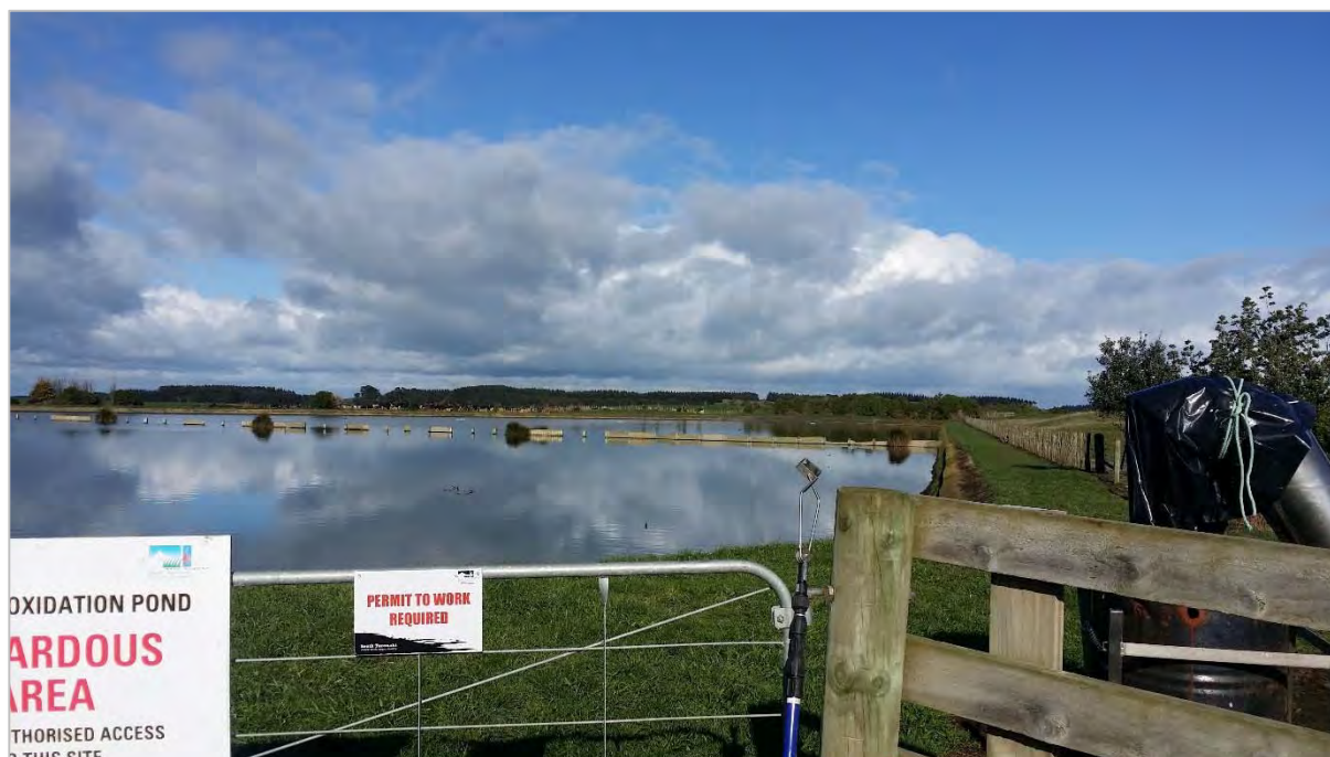
Photo 7 Waverley WWTP, August 2016
