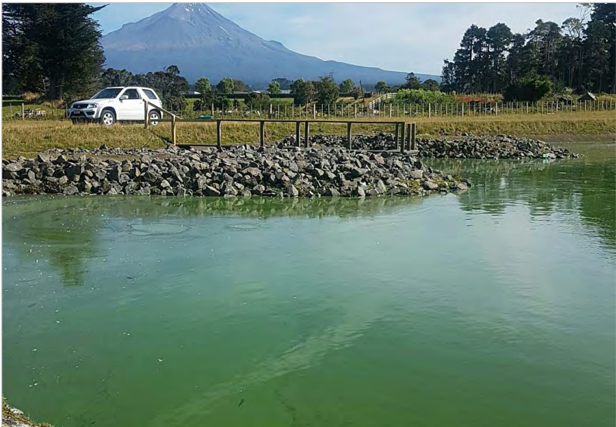
Photo 1 Kaponga WWTP, February 2017
