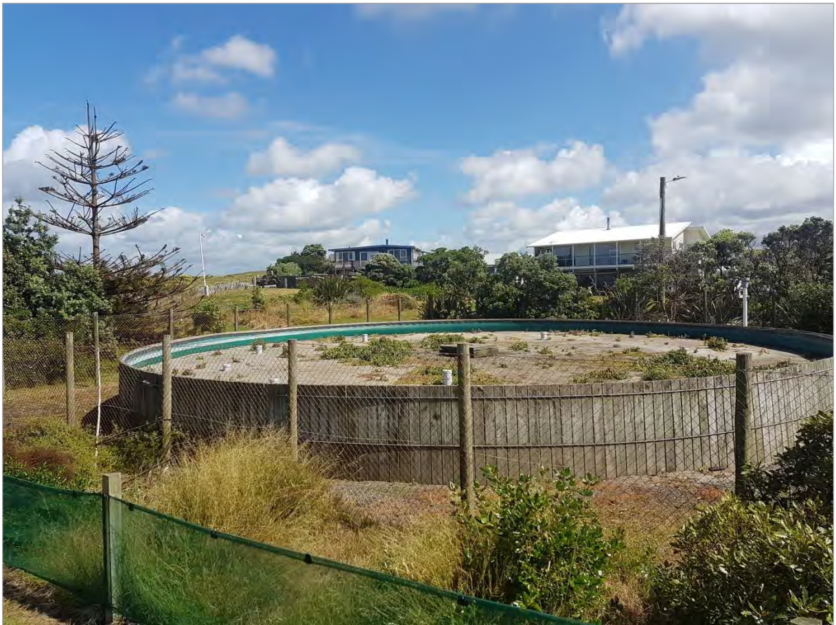
Photo 1 Moderate weed growth on the western filter bed at Wai-inu Beach Settlement (13 December 2016)
