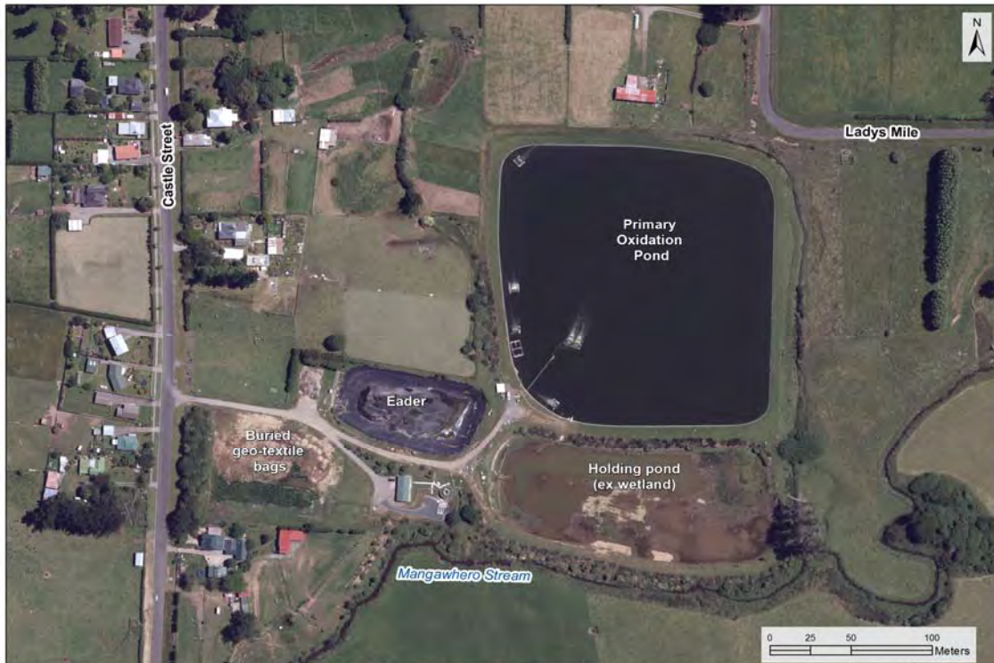
Figure 2 Aerial view of the Eltham WWTW
