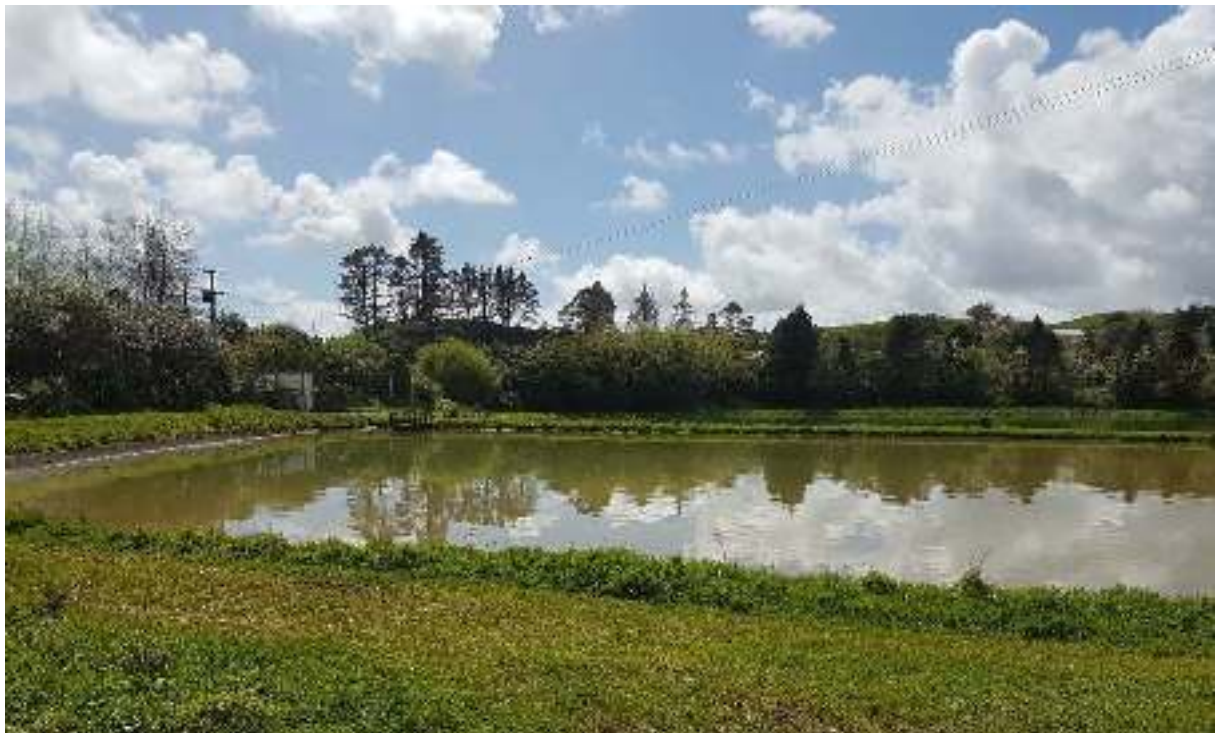
Photo 3 The Inglewood WWTP main pond
