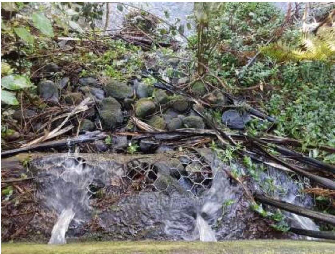
Photo 5 Overflow discharge from Inglewood WWTP entering the Kurapete Stream, 25 July 2017
