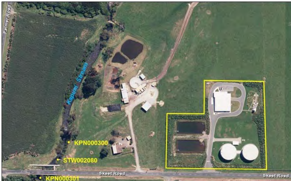
Figure 3 Aerial photo showing locations of the Kapuni WTP, and relevant sampling sites
