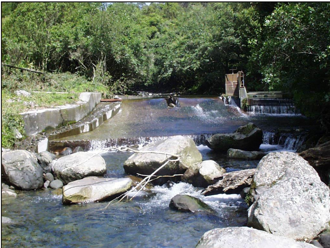
Photograph 1 Ngatoro Stream weir
