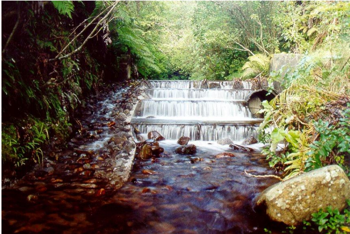
Figure 1 Wairau Stream weir and fish pass
