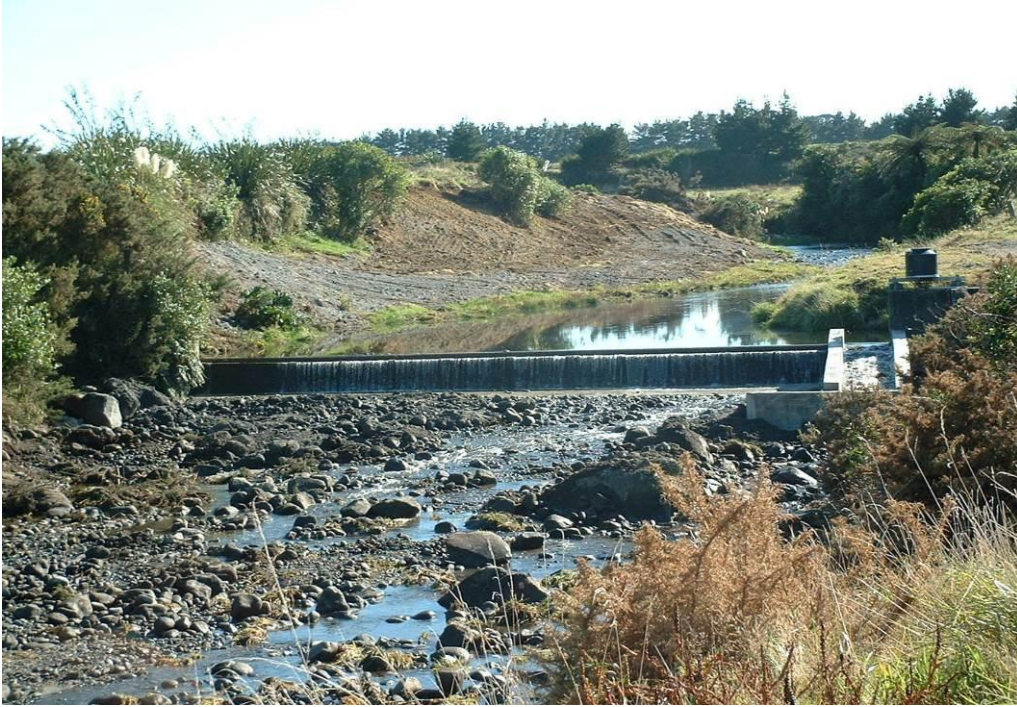
Photo 1 Oaonui Water Supply weir post installation (April 2002) of new fish pass and repairs to splash pad
