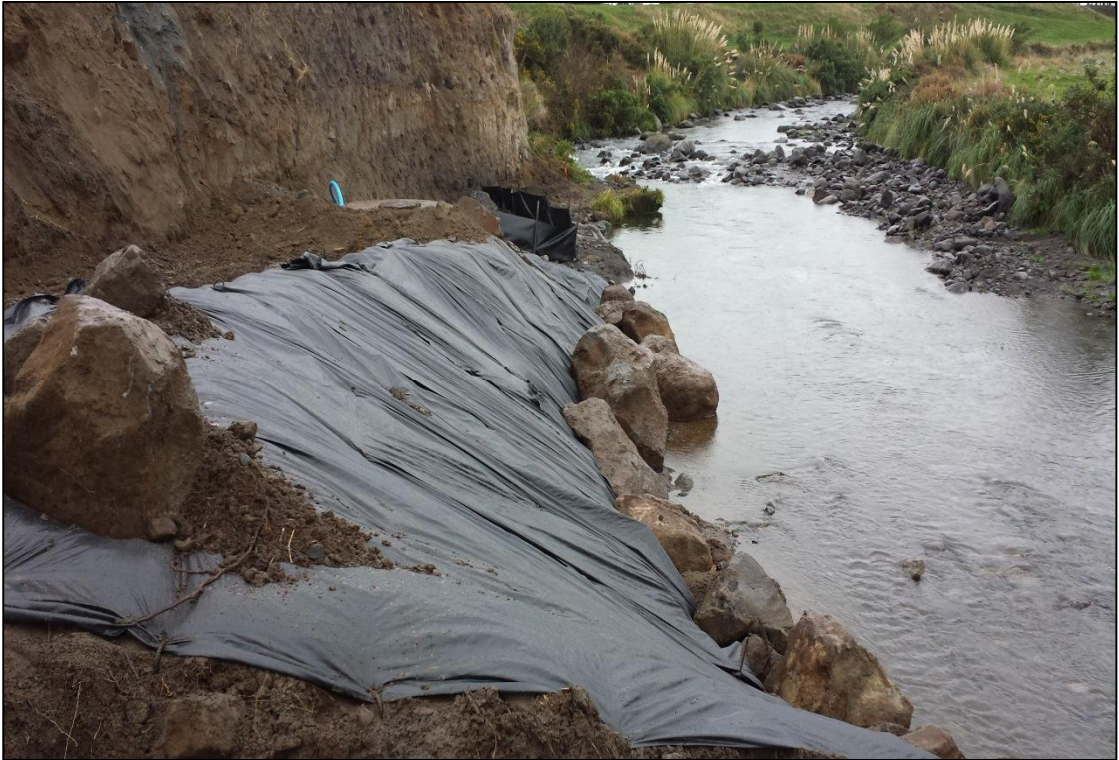
Photograph 6 Silt controls at the Opunake WTP intake installation
