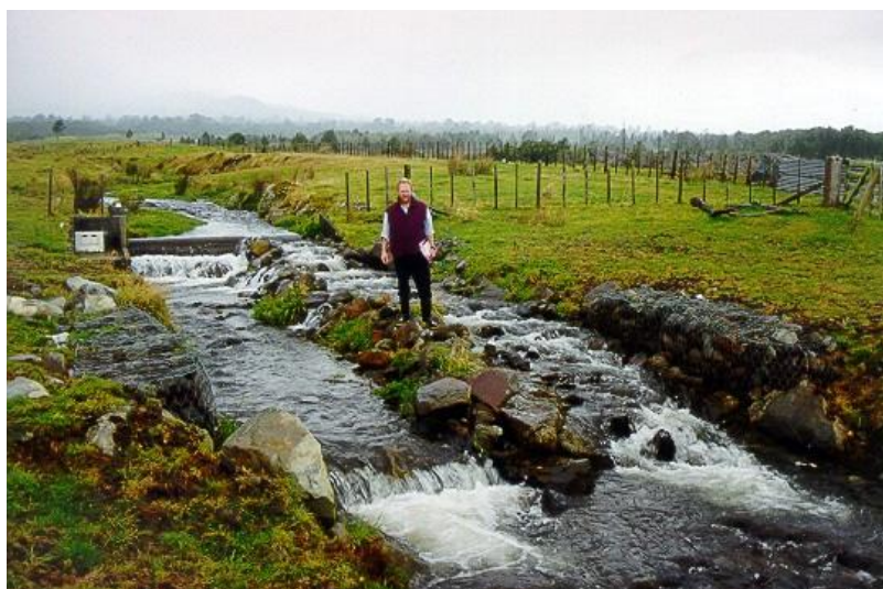
Photo 1 Cold Stream weir and fish pass
