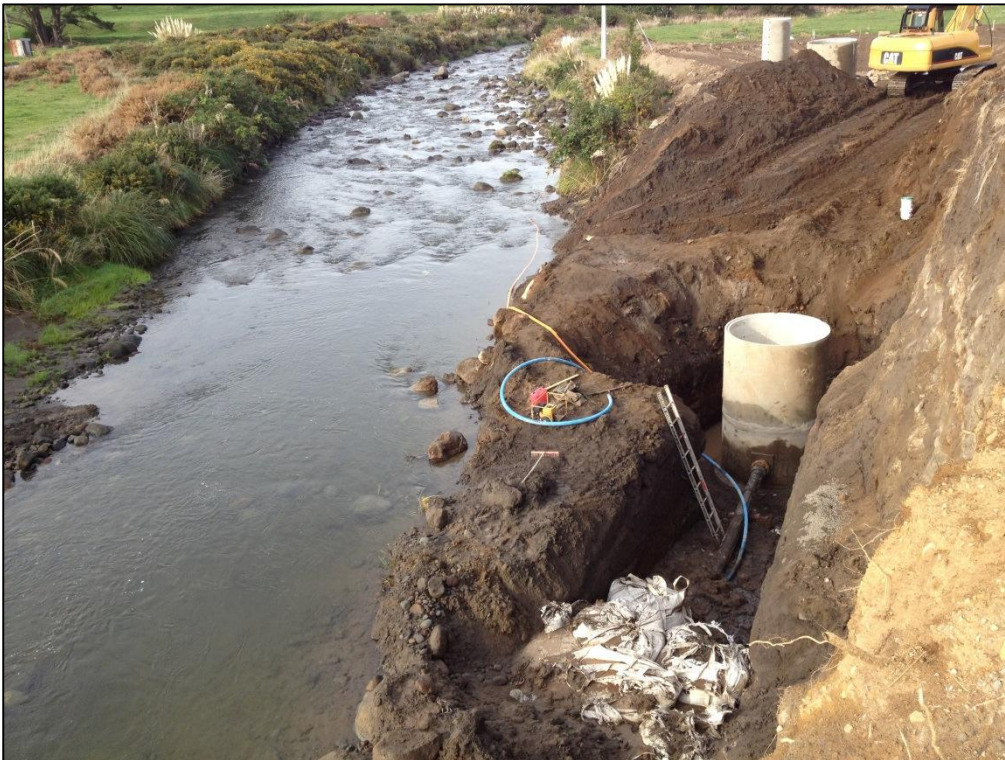
Photograph 5 Wet well and intake line installation at the Opunake WTP
