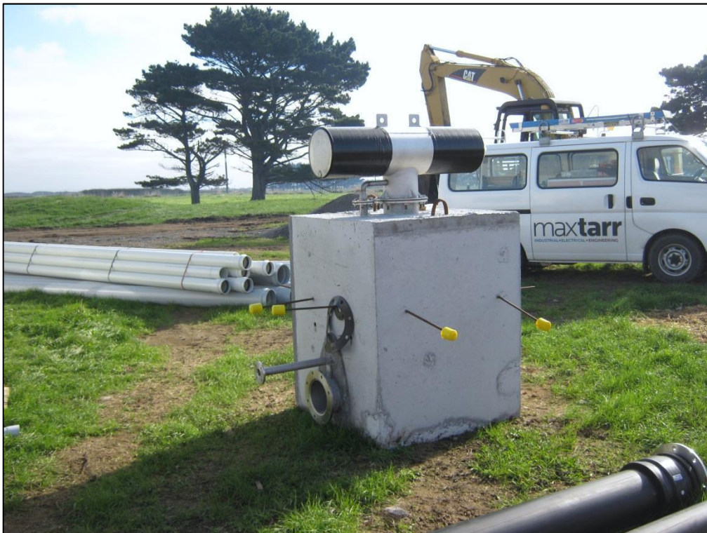
Photograph 4 Opunake WTP intake structure prior to installation
