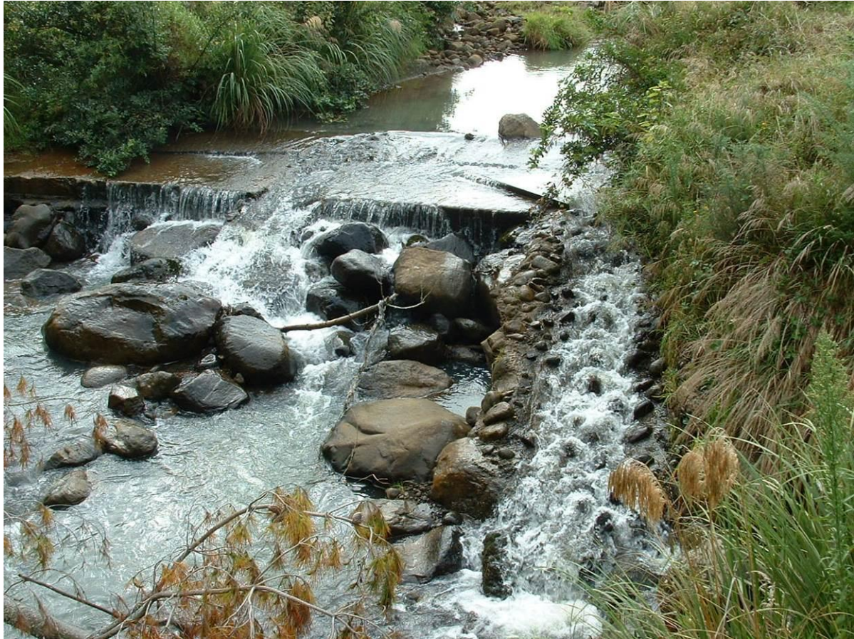
Photo 1 STDC weir, new fish pass (right of photo) and old fish pass (left of photo) in the Mangawhero Stream
