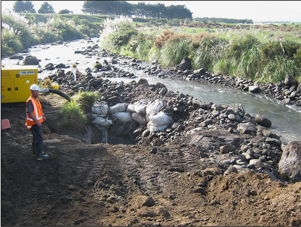
Photograph 3 Cofferdam on the Waiaua Stream for Opunake WTP intake installation
