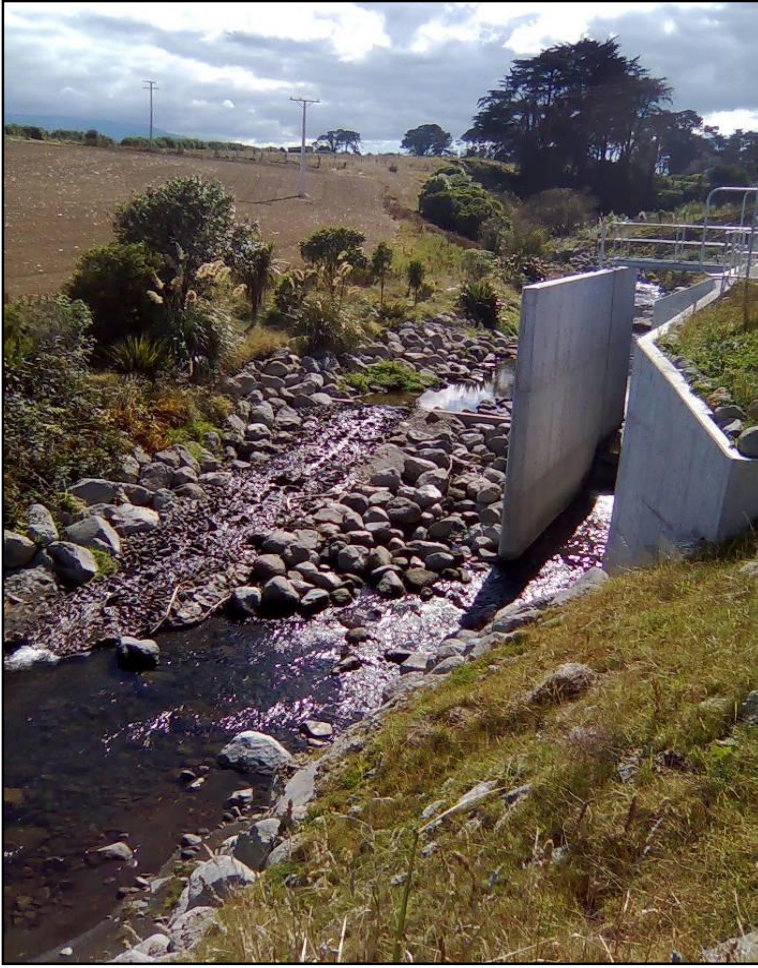
Photograph 2 Kapuni WTP intake and fishpass on the Kapuni Stream
