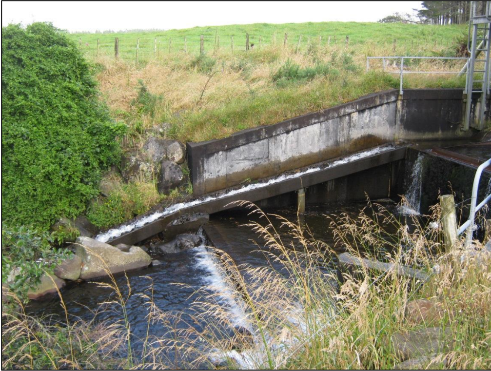
Photograph 8 Fish pass at Mangawhero-iti weir
