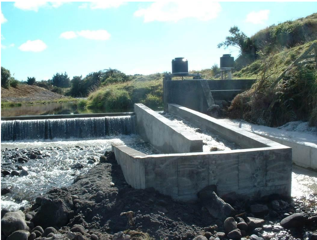
Photo 2 The operating fish pass (April 2002) at the Oaonui Water Supply weir
