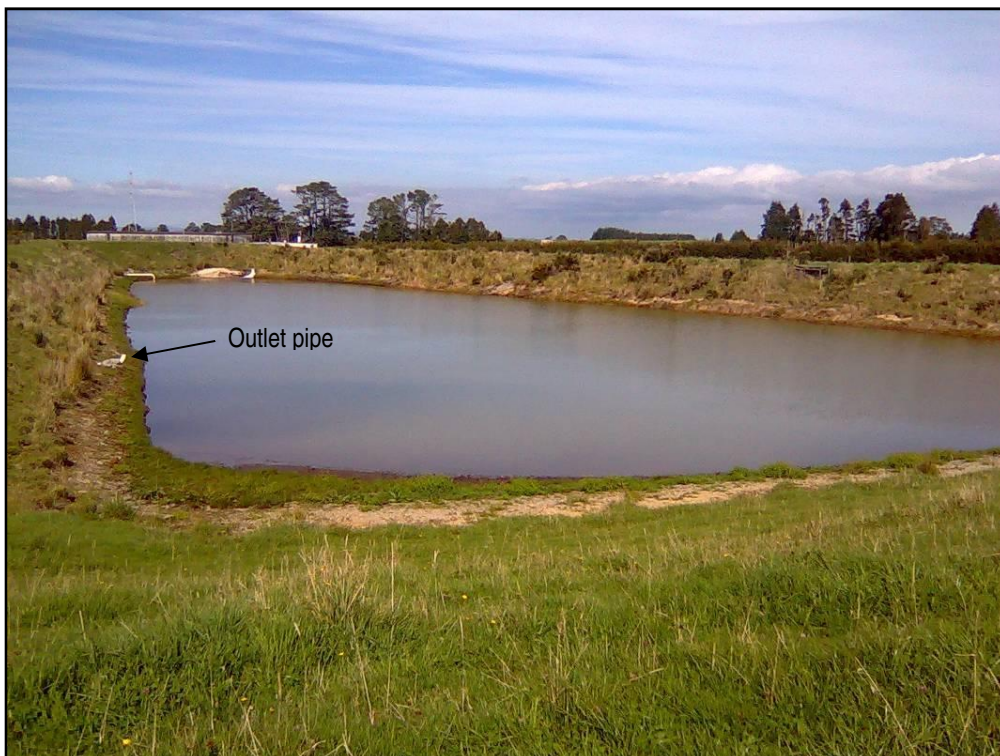
Photograph 1 Stratford WTP settling pond, showing location of outlet pipe
