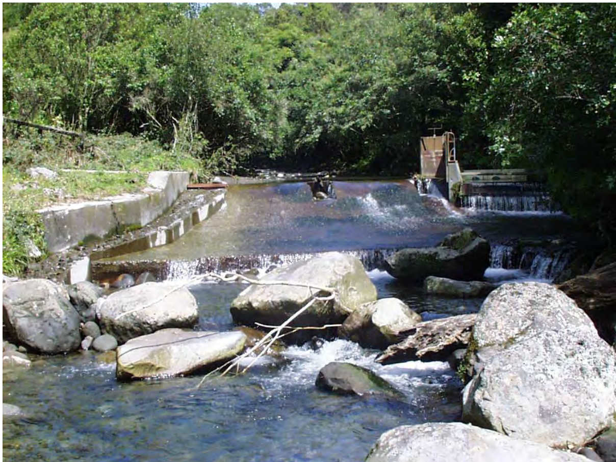
Figure 2 Ngatoro Stream weir and fish pass
