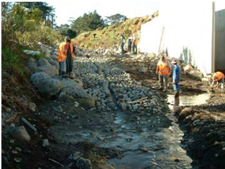
Photo 1 The STDC fish pass being installed September 2009
