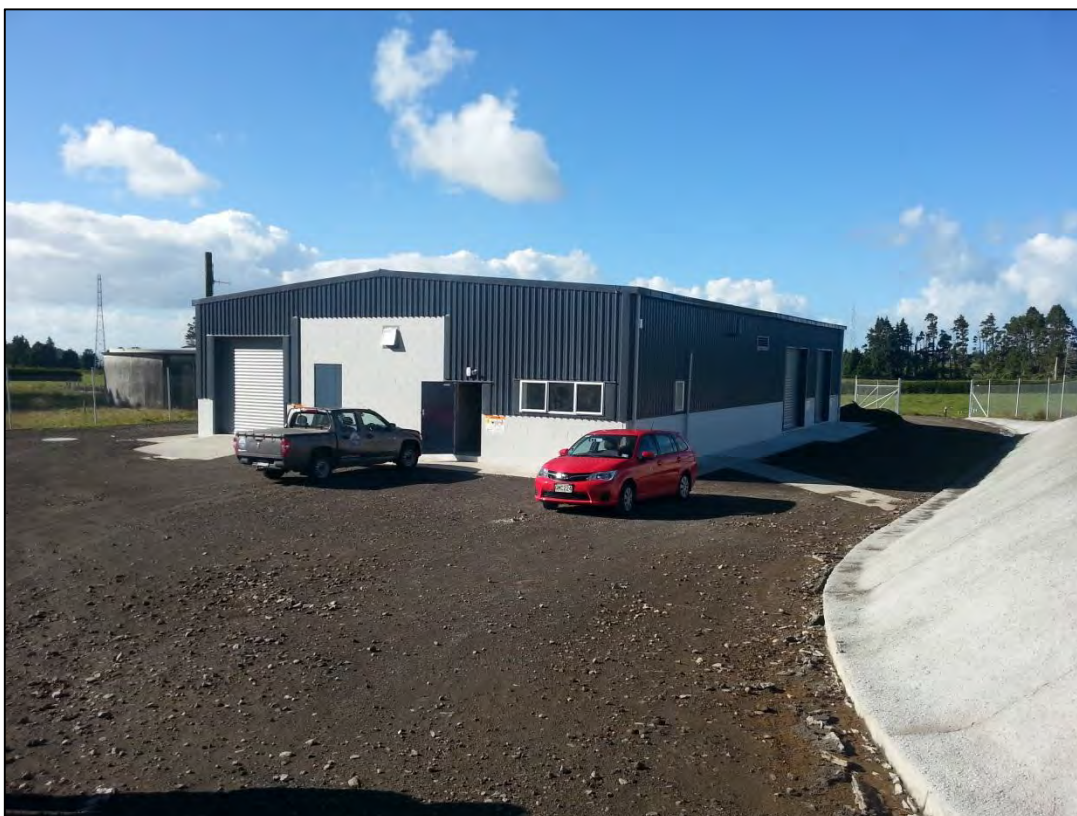
Photo 1 New Stratford WTP
